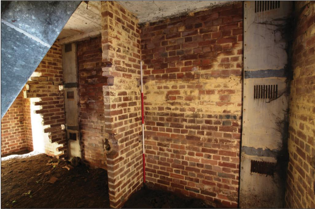
Plate 43: Detail of typical bunk bed bays (bunks removed) in sleeping shelter showing heating vents
