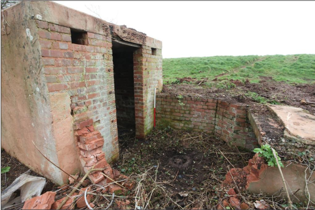
Plate 35: Defence post 45a exterior showing gun-pit, magazine and shelter entrance
