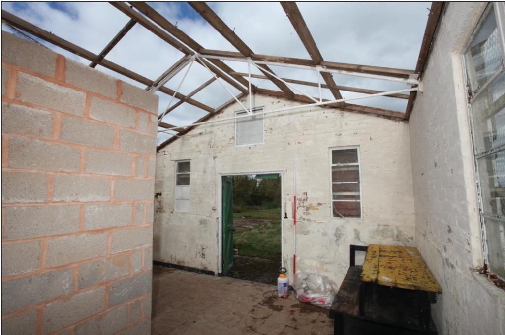
Plate 28: Interior of Flight offices 'DK' showing roof truss and sheet purlins
