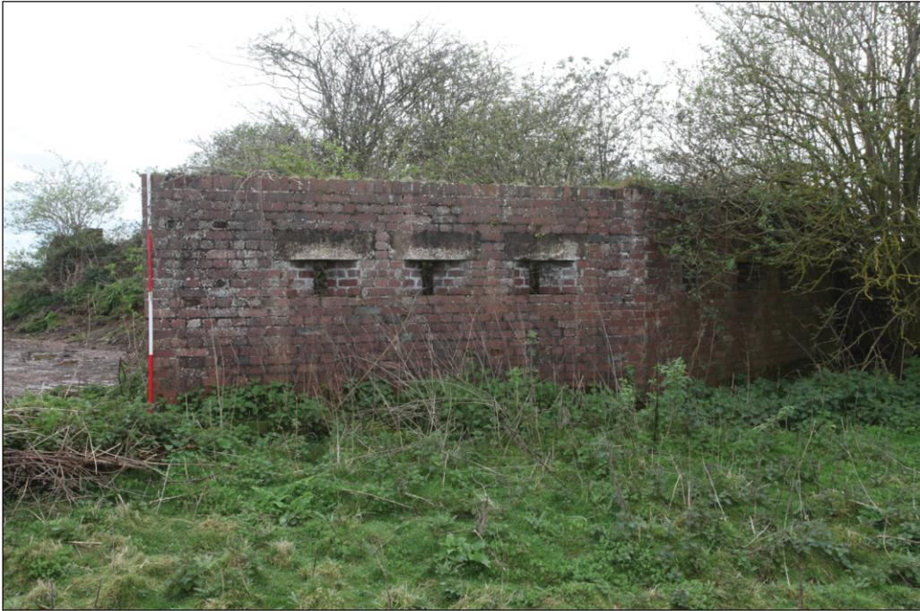
Plate 17: Defended wall with loop holes fighter pen 81
