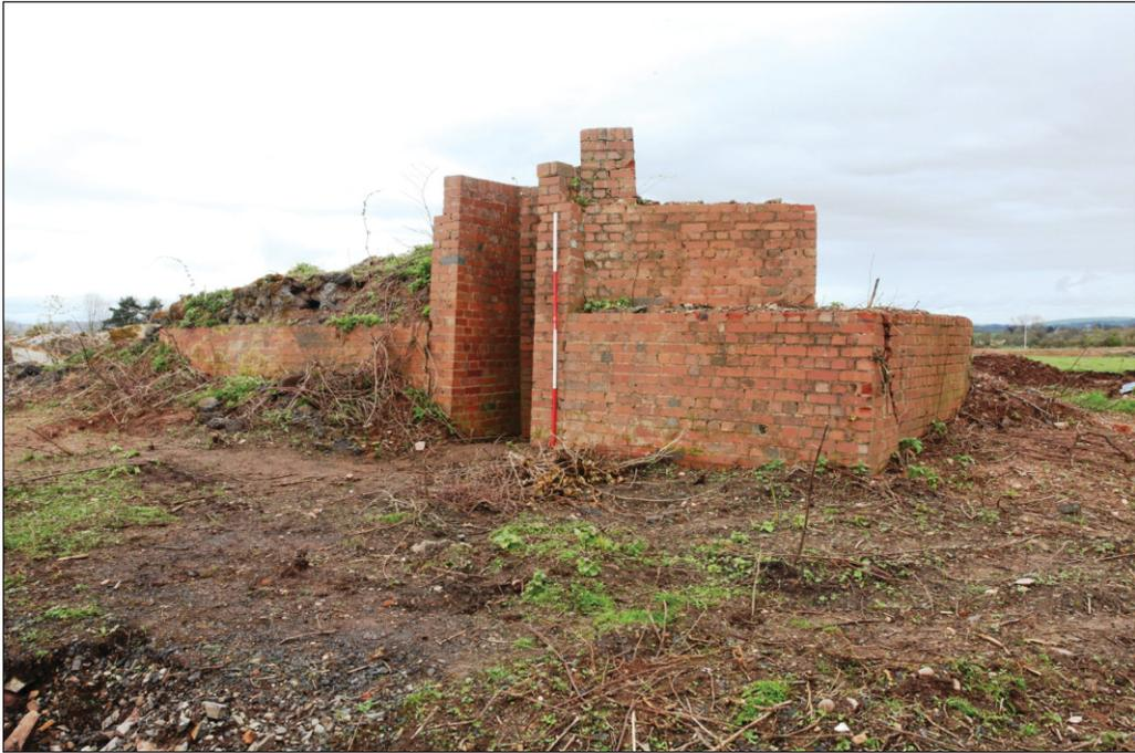
Plate 11: Shelter entrance to pen 90. Note 'sand' bags on top of central wall
