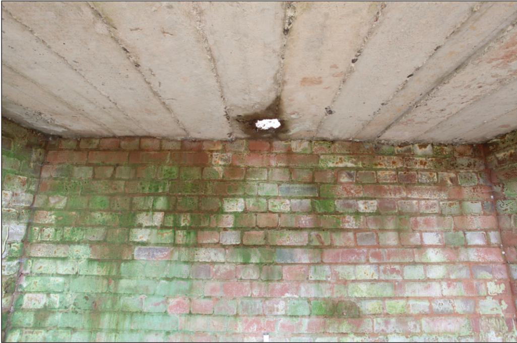
Plate 37: Defence post 45a interior roof showing stove pipe aperture
