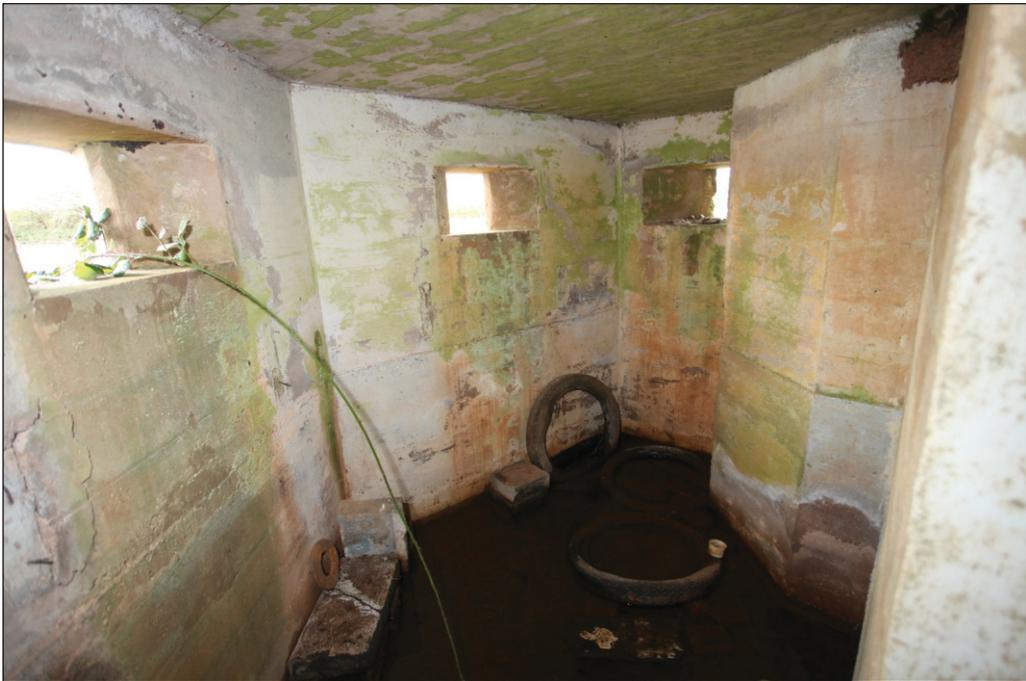
Plate 40: Defence post 32 interior showing embrasures and blast protection wall
