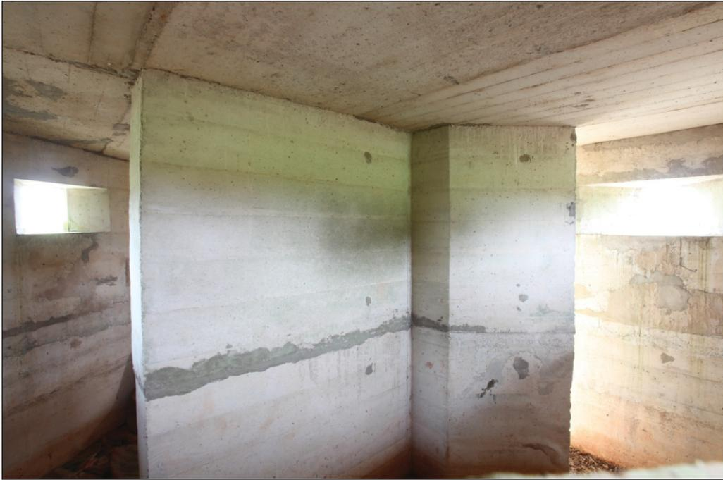
Plate 33: Defence post 45 interior blast protection wall
