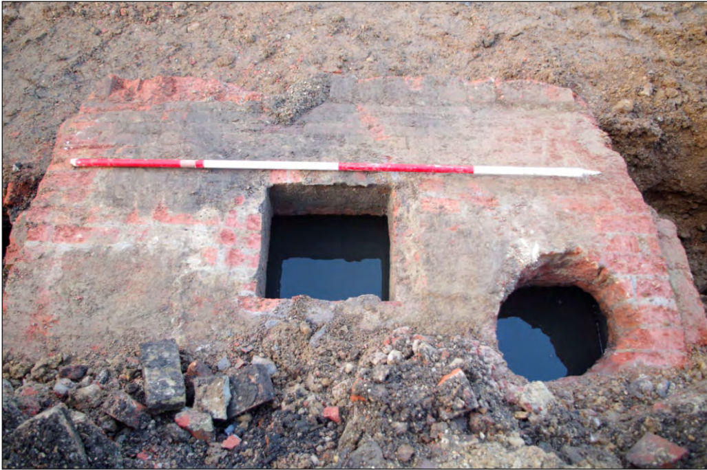
Plate 5: Plan view of modern interception tank 409, viewed from the north-west. Scales = 1 m and 2 m
