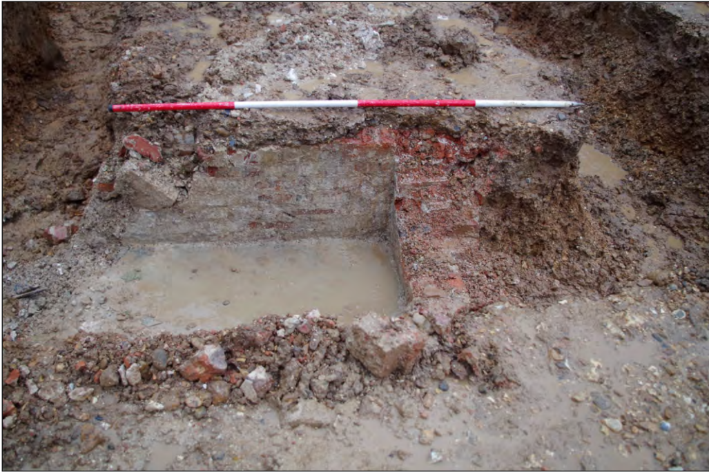
Plate 7: Modern wall with concrete base 406, viewed from the east. Scale = 2 m
