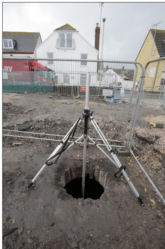
Plate 2: Access hole and scanner tripod
