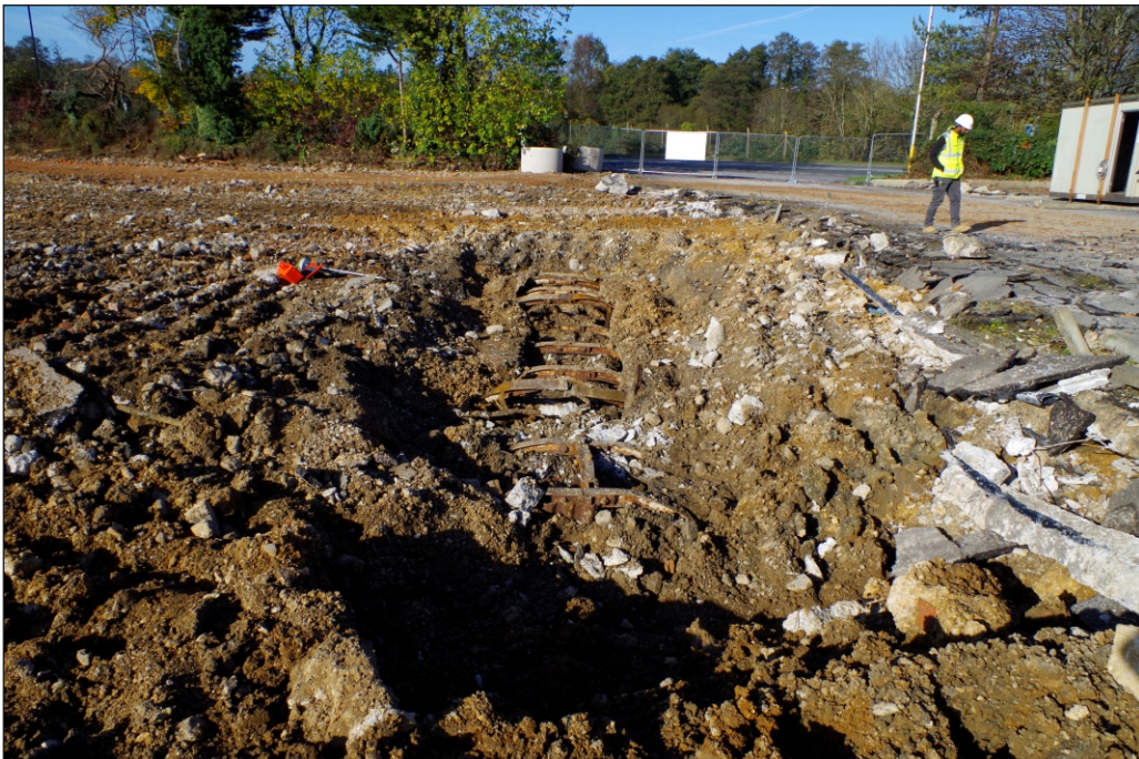
Plate 2: Example of Anderson shelter showing construction and rubble backfill (viewed from the south-west)
