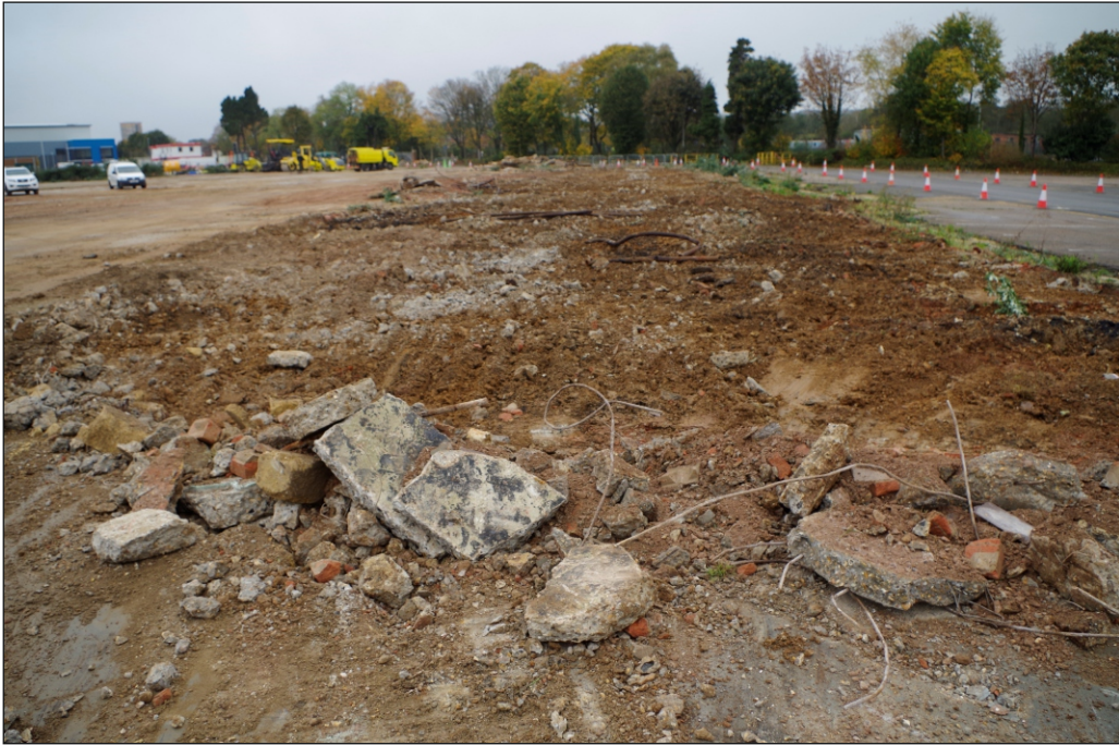
Plate 1: Concrete slab during removal
