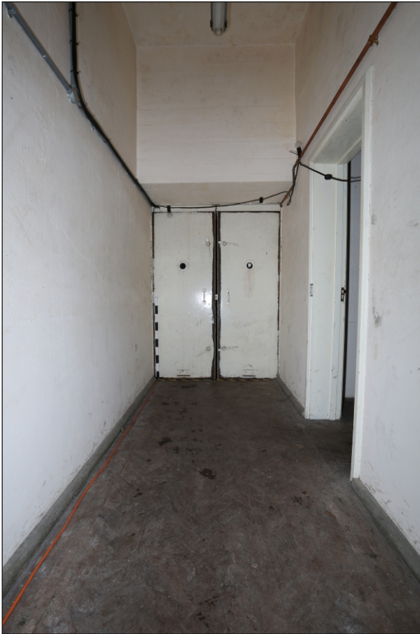
Plate 13: Corridor D1 showing sealed doors and parquet flooring
