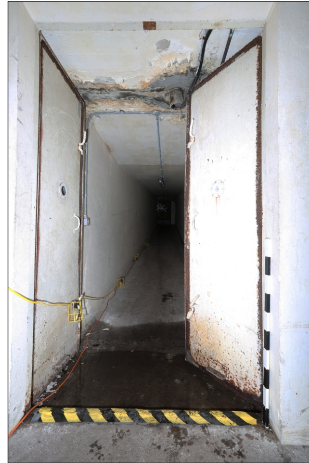
Plate 6: Sealable doors at base of entrance passage A2
