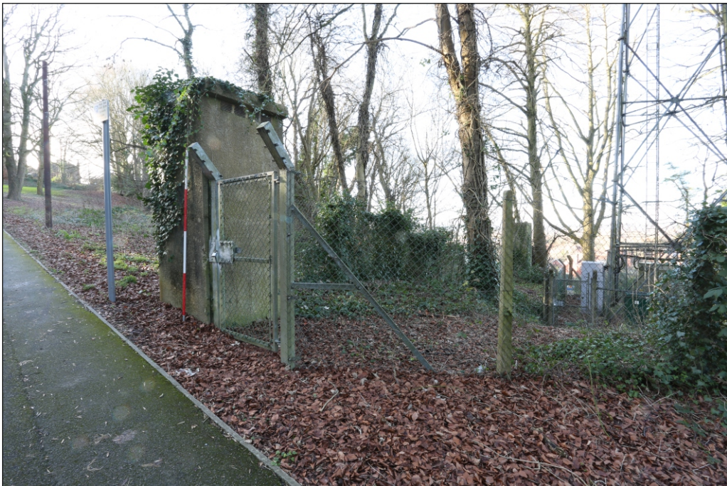
Plate 36: South vent shaft
