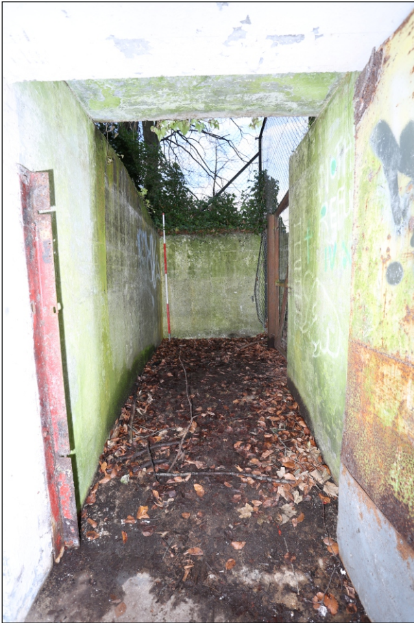
Plate 3: Entrance path A1 viewed from main doorway
