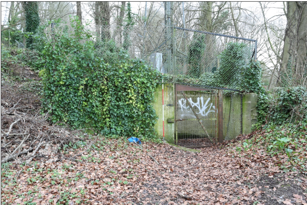
Plate 2: Fenced and gated Bunker entrance A1
