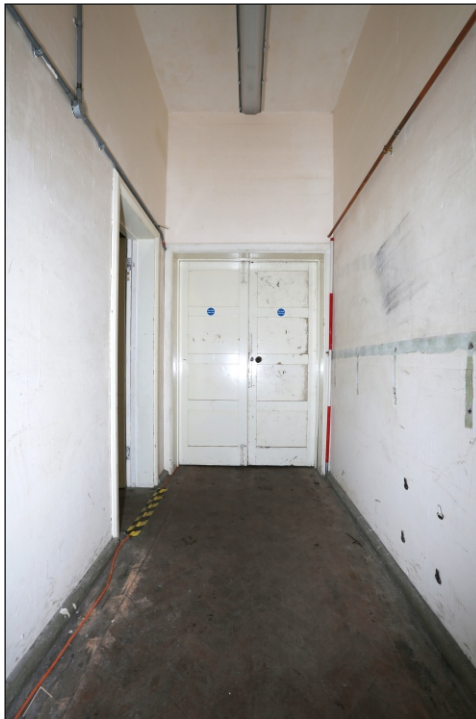
Plate 15: Corridor D2 showing west side of doors and shelving scar to right
