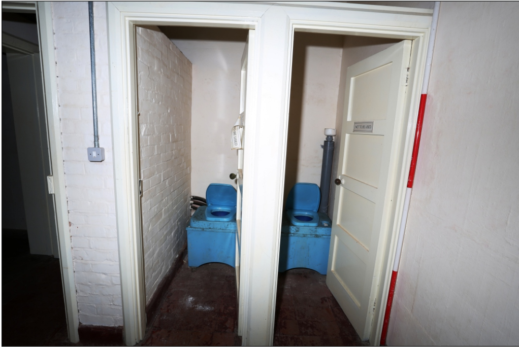
Plate 31: Toilet N cubicles fitted with plastic toilets
