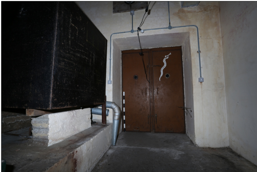
Plate 12: Generator room C inside face of doors original colour scheme
