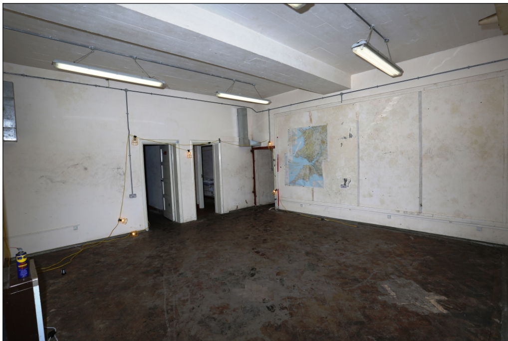
Plate 22: Control room I showing fibre board covered wall and access to escape tunnel
