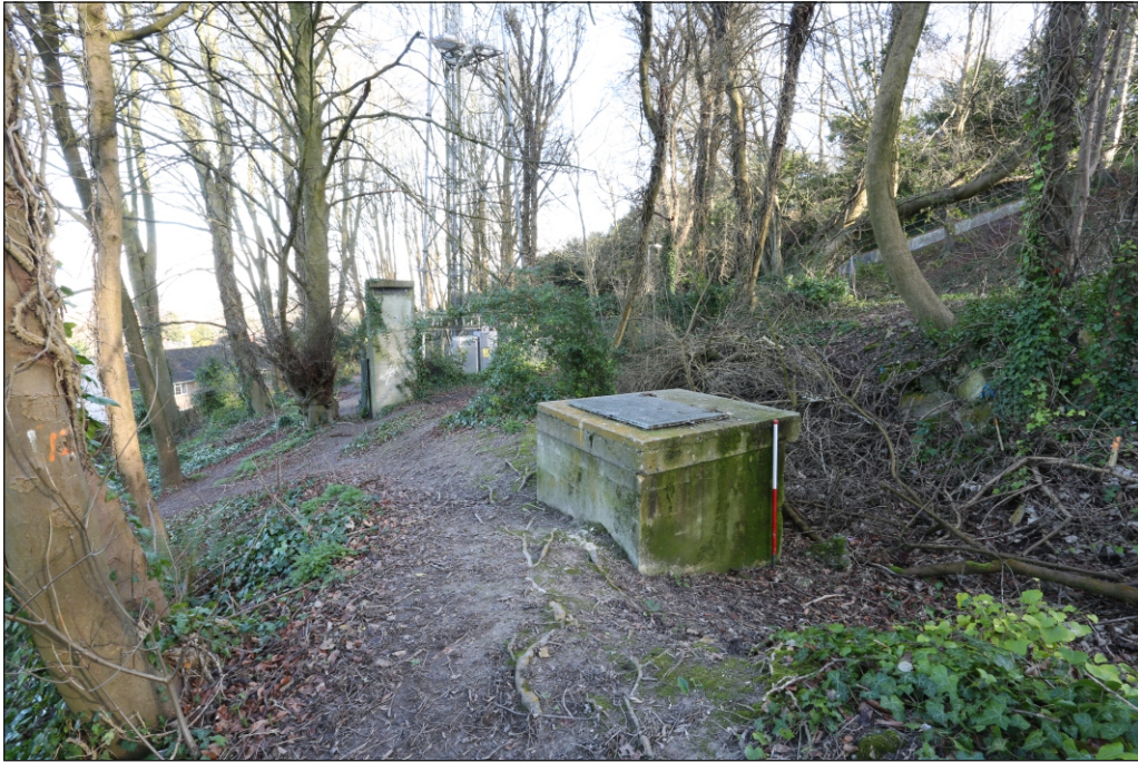
Plate 35: Top of escape hatch shaft north-west
