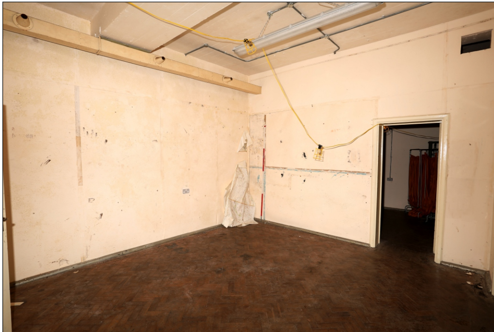
Plate 21: Situation room H showing fibre board wall and air ducting vents
