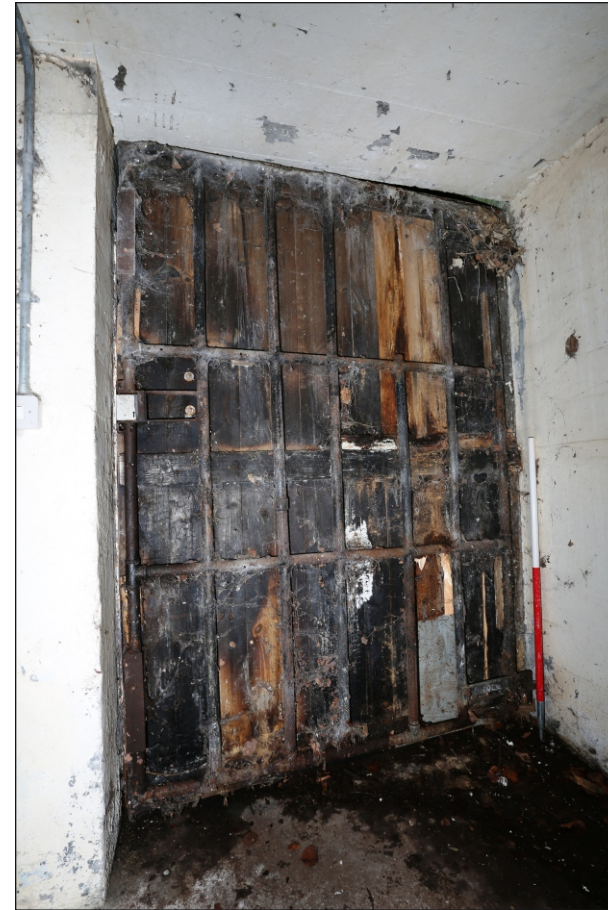
Plate 4: Steel pipe entrance gate viewed from interior
