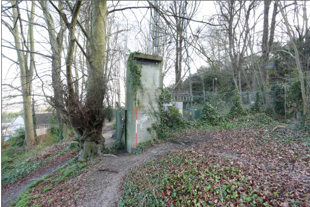
Plate 34: North-east high exhaust vent with cover grills
