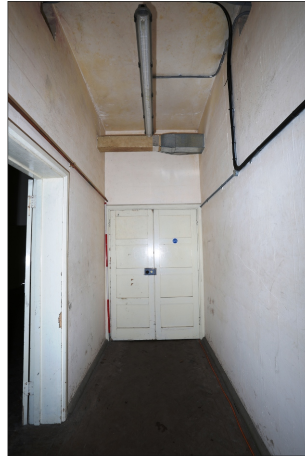
Plate 14: Corridor D1 showing wooden doors at west end
