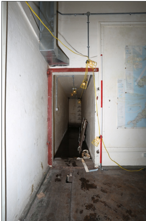
Plate 25: Entrance to escape passage K showing removed steel door
