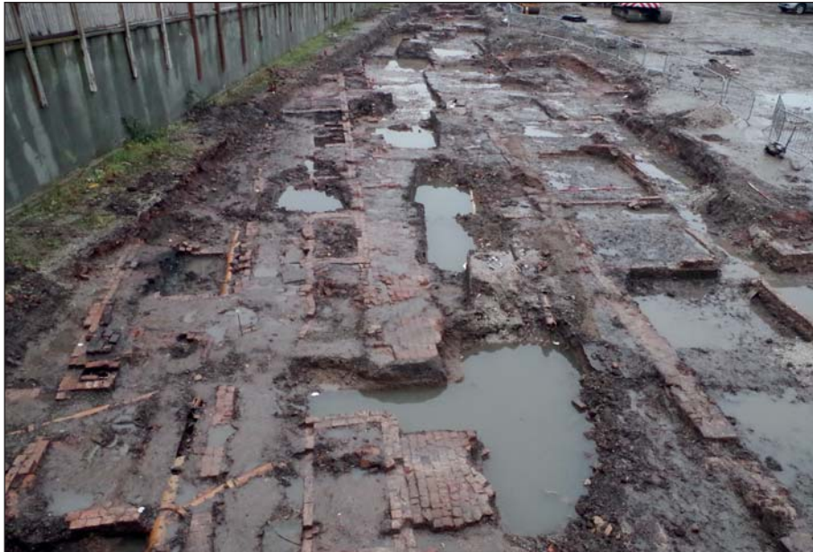
Plate 14: Terraced housing in north-east of site. Wall 25 dividing outhouses runs approximately down the centre of the shot, with Fosbrook Street yards to the left and Albert Terrace yards to the right. View from north
