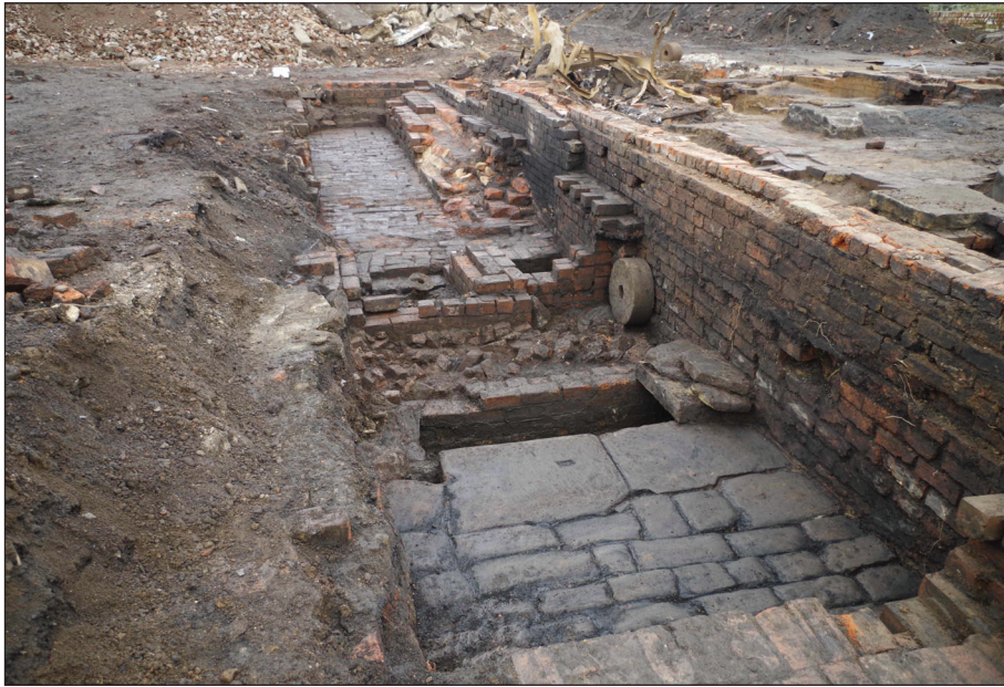
Plate 7: Phase one boiler house showing internal features, facing south-east.
