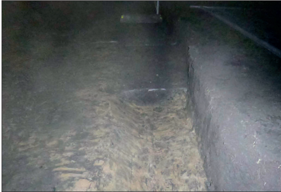
Figure 4: Ditch 304, view from the south-east
