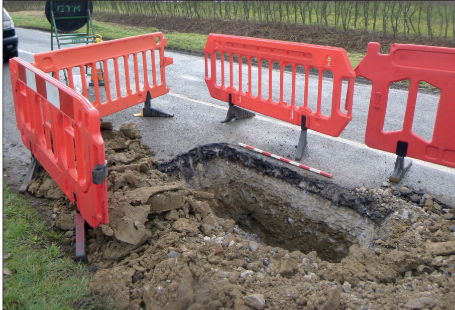
Figure 6: Trench 32, view from north-east (1 m scale)
