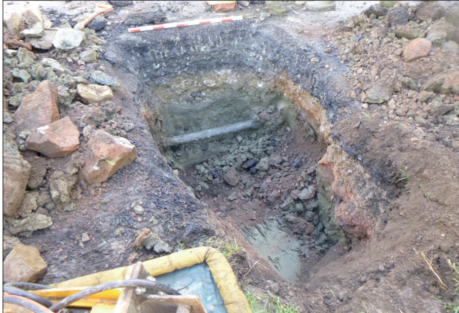
Figure 4: Trench 36, view from south (1 m scale)
