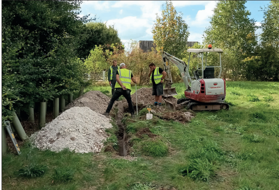
Figure 7: General view of the excavation of Test Pit 3 from the west
