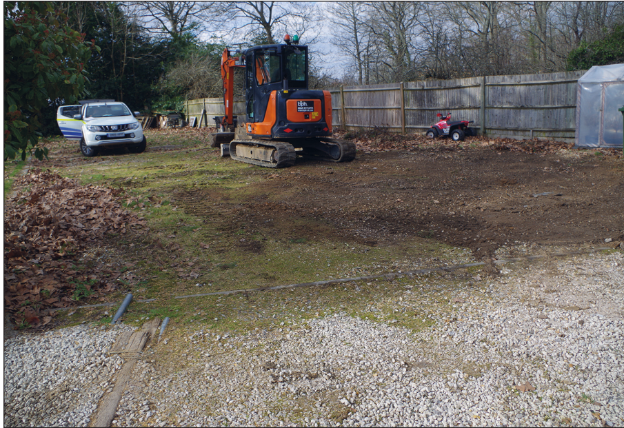
Figure 2: View of site from the east, trench backfilled.
