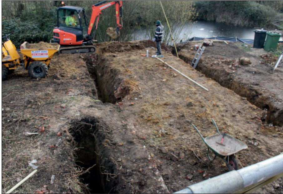
Figure 2: Trench 1 from the west
