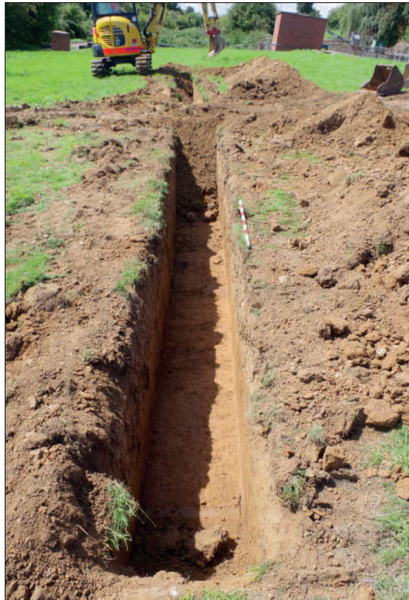
Figure 5: General shot of Trench 2. View from north east
