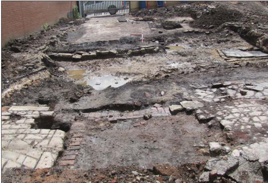
Plate 66: Overview of Area K from the north
