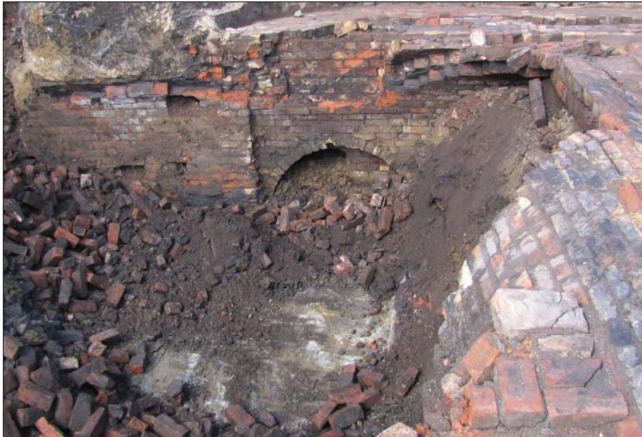
Plate 50: Opening in west side of cellar 2041 (removed) seen during watching brief from the east Vaulting 2074 is visible at right of shot
