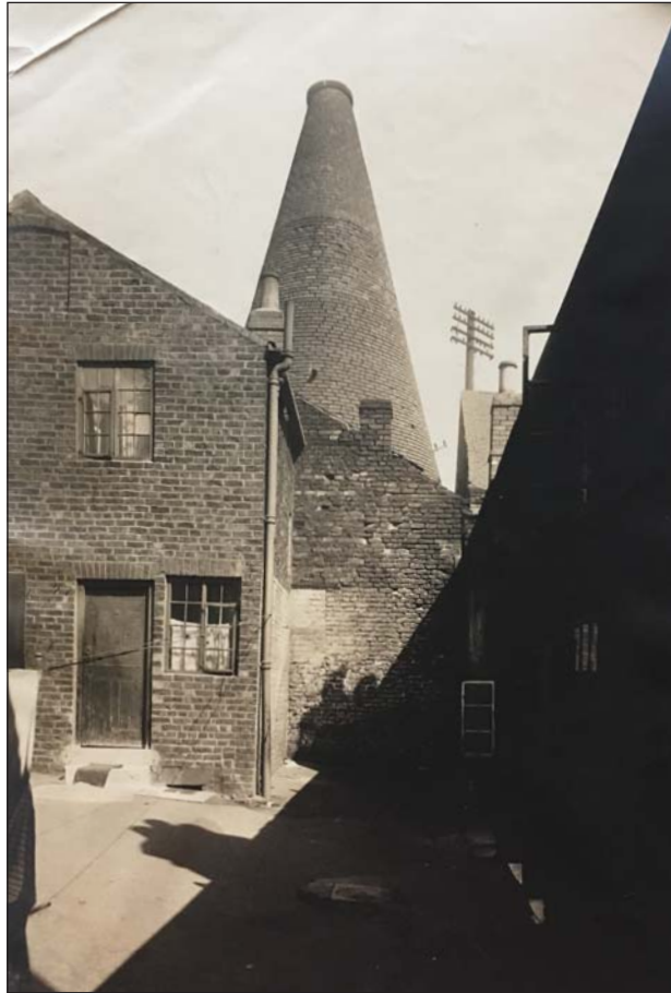
Plate 1: Cementation furnaces (not the same as those excavated) at Hollis Croft from Footprint Sheffield archive. View probably from the east
