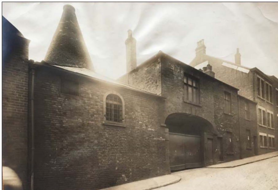
Plate 2: Cementation furnaces (not the same as those excavated) at Hollis Croft from Footprint Sheffield archive. View probably from the north-east
