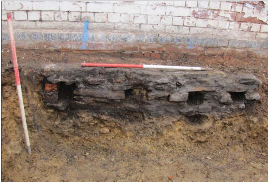
Plate 8: Wall 3006 with sockets for wooden floor joists from the east
