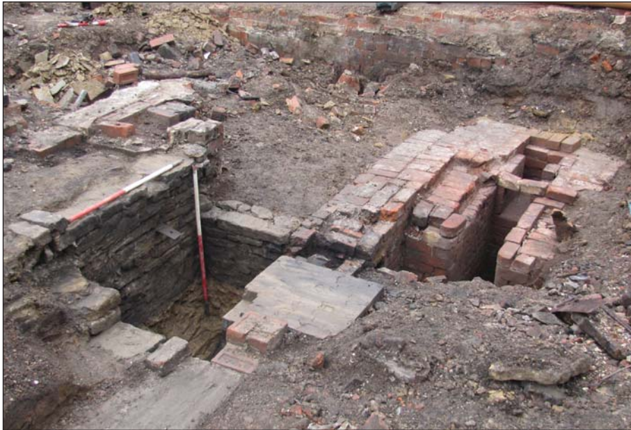
Plate 25: Wall 1745 and associated structures with crucible furnace 1747–1750 in background from the north-west
