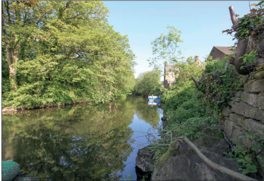
Figure 3: River wall, view from the south-east
