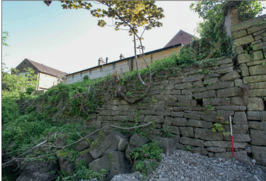
Figure 6: Southern section of the river wall, view from the south
