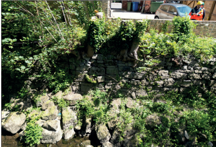
Figure 10: Two medium-sized trees and vegetation growth at the middle section of the river wall, view from the south-west
