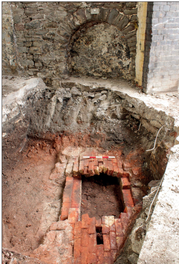
Figure 56: Brick flue (1054, group 1087) in north corner of coal store, looking west. Scale: 1 m (photograph by C. Mason).
