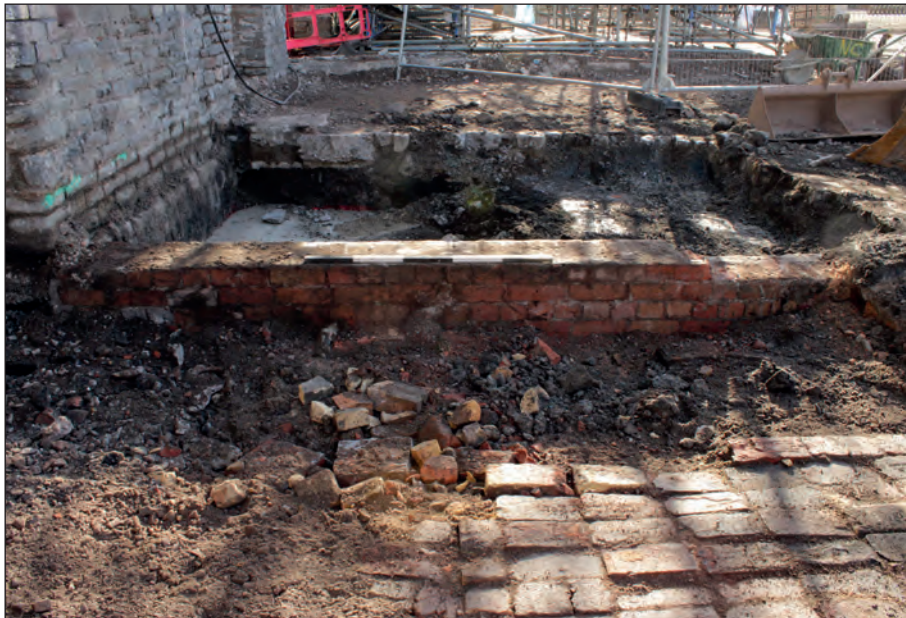
Figure 97: Brick and concrete ramp structure (group 2048), looking south-east. Scale: 1 m (photograph by C. Sabato).
