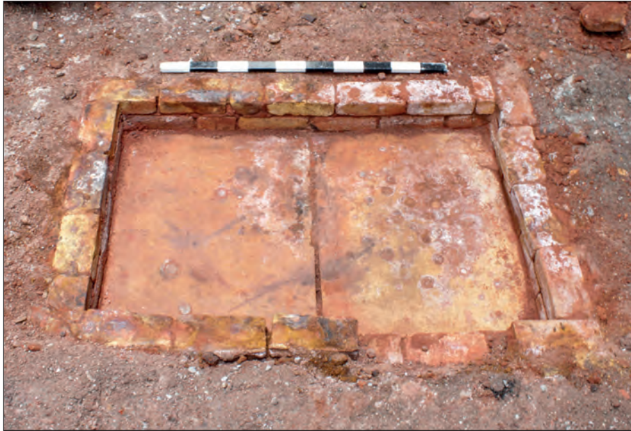
Figure 68: Interlocking fireclay slabs over access hole into underground flue (group 1084) in coal store, looking north-east. Scale: 1 m (photograph by C. Mason).
