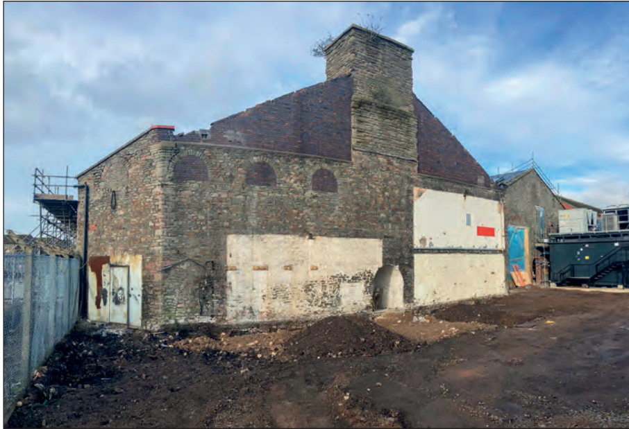
Figure 32: North-east elevation of the coal store (photograph by C. Mason).
