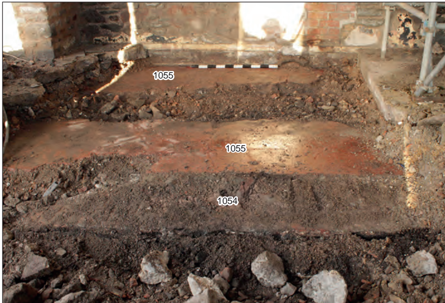
Figure 65: Wall 1054 and red concrete floor 1055 in west corner of coal store, looking north-west. Scale: 1 m (photograph by C. Mason).
