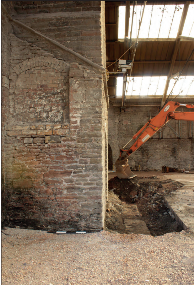
Figure 46: Stone wall foundation (1048, group 1085) and upstanding chimney in coal store, showing line of coping stones and opening into north-west side of chimney. Looking south-east. Scale: 1 m (photograph by C. Mason).
