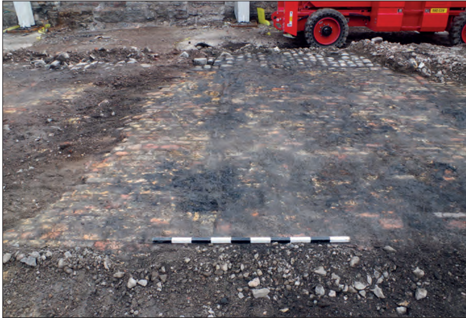
Figure 76: Firebrick and sandstone sett floor (group 1082) on the south-east side of the coal store, looking south-east. Scale: 1 m (photograph by C. Sabato).
