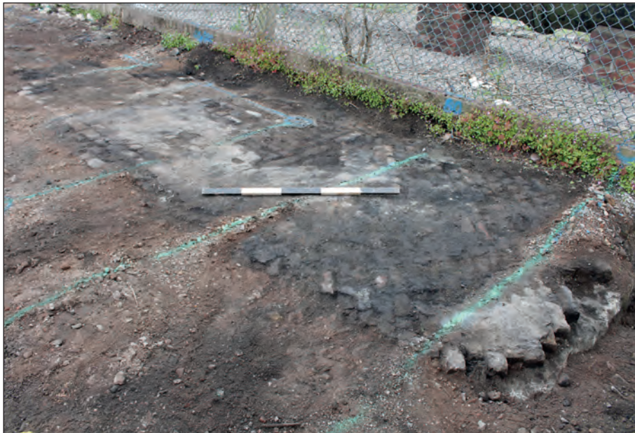
Figure 103: Brick floor (group 4082) to the north-east of the retort house, looking east. Scale: 1 m (photograph by L. Jervis).
