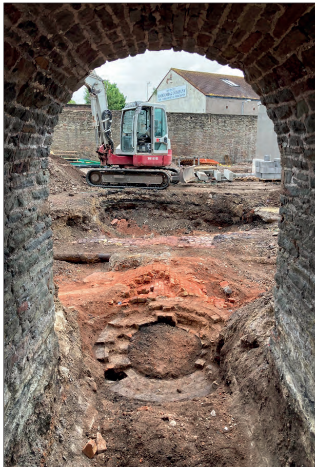
Figure 63: Arched doorway under the coal store chimney, looking north-east towards well 4069 and flue system 4083 (photograph by C. Mason).
