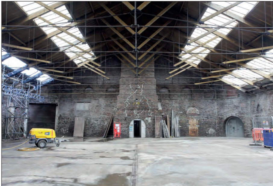
Figure 35: Interior of coal store, looking north-east (photograph by C. Mason).
