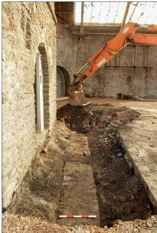
Figure 45: Stone wall foundation (1048, group 1085) and upstanding chimney in coal store, looking south-east. Scale: 0.5 m (photograph by C. Mason).
