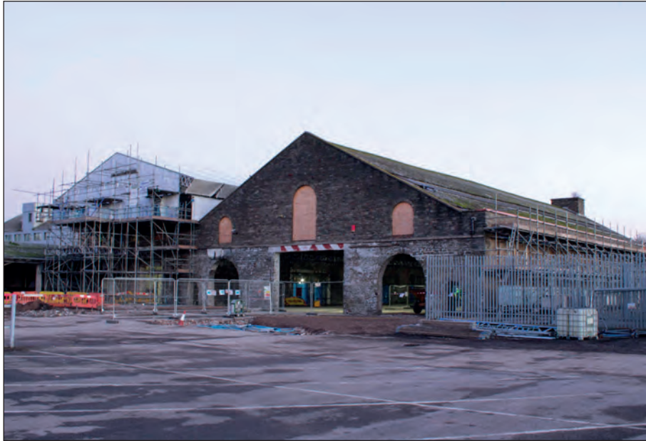
Figure 30: Coal store and retort house, looking north (photograph by C. Mason).
