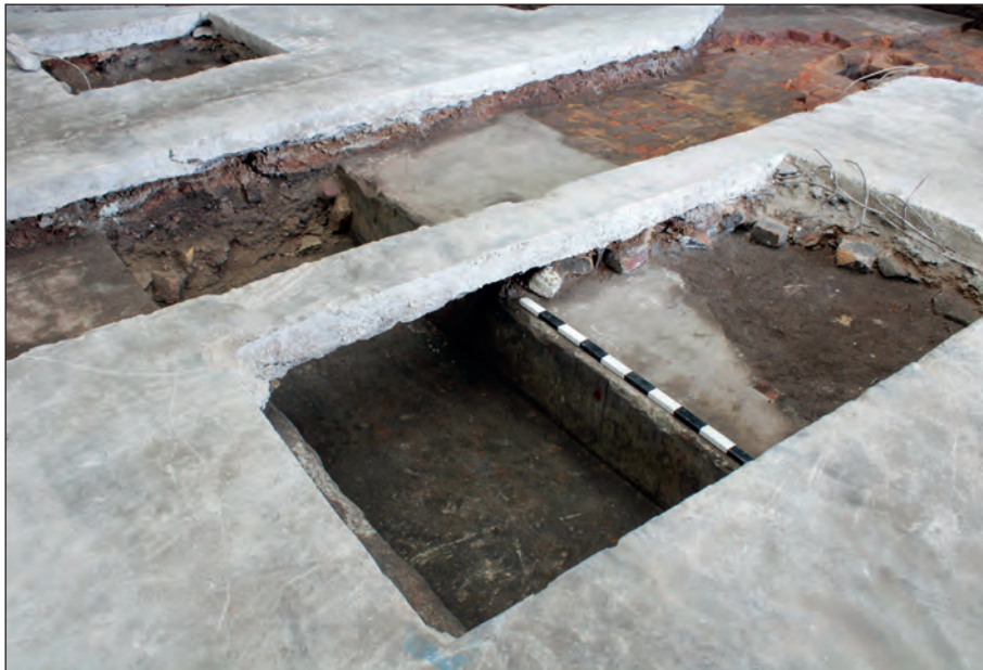
Figure 93: Concrete trough of cooker incinerator (group 3060) in the north-west range of the retort house, looking east. Scale: 1 m (photograph by C. Hambleton).
