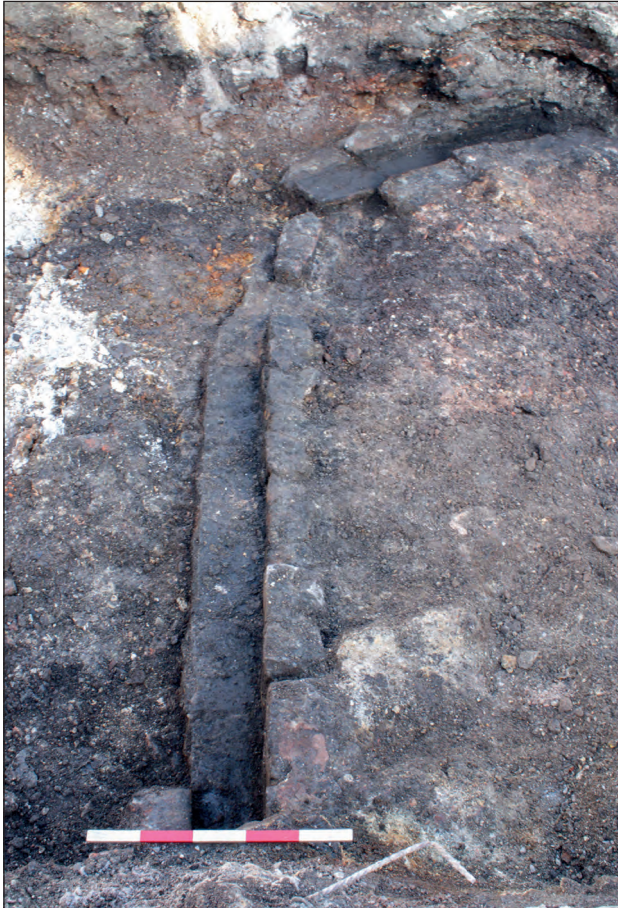
Figure 80: Brick- and stone-lined drain (group 1088), looking north-east. Scale: 0.5 m (photograph by C. Sabato).
