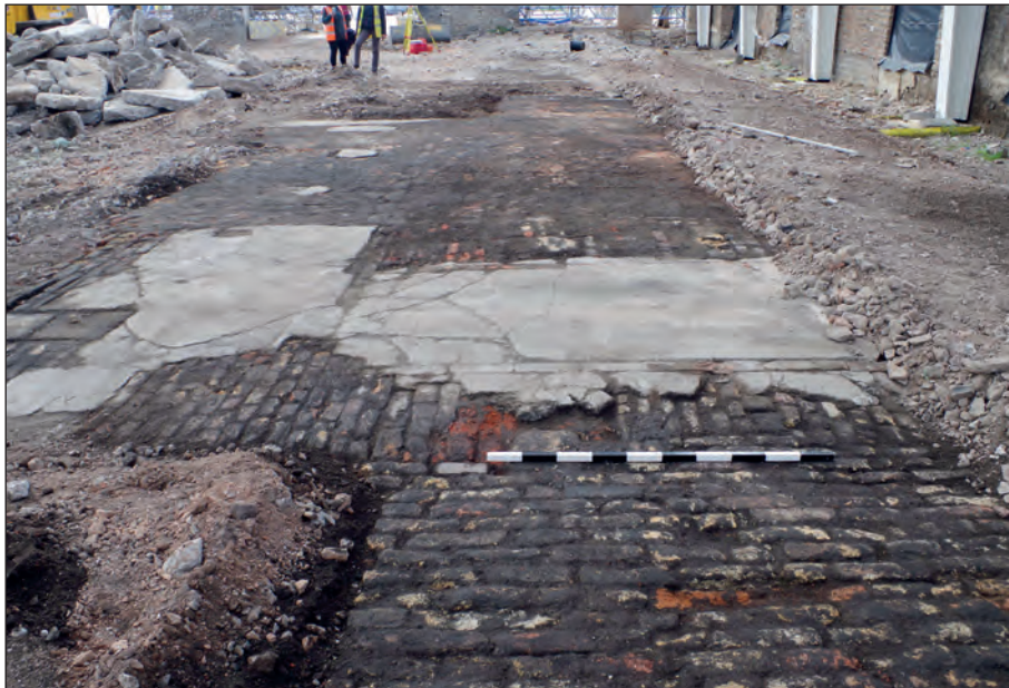
Figure 79: Sandstone sett floor (group 1082) and modern concrete repairs (group 1086). Scale: 1 m (photograph by C. Sabato).
