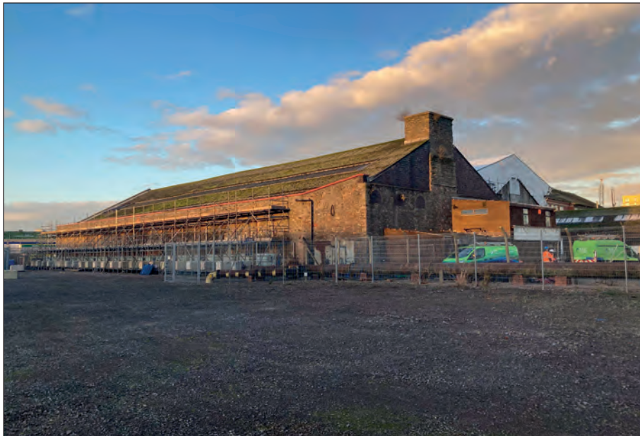
Figure 31: Coal store, looking west (photograph by C. Mason).
