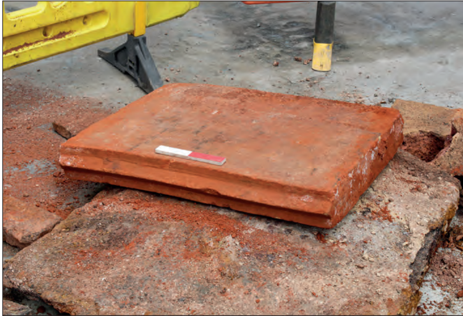
Figure 70: Detail of fireclay capping slab showing tongue and groove moulding on edge. Scale: 0.2 m (photograph by C. Mason).
