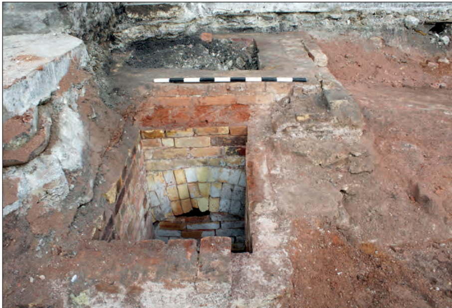
Figure 73: Openings at north end of flue (group 1084) in coal store, looking north-east (photograph by C. Sabato).
