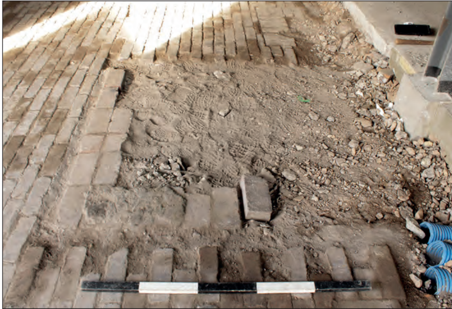
Figure 94: Brickwork at south-west end of cooker incinerator (group 3060) and brick floor (group 3055) in the north-west range of the retort house, looking north-west. Scale: 1 m (photograph by C. Sabato).
