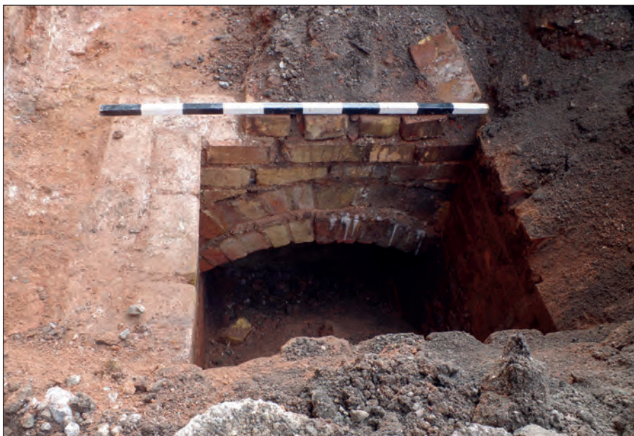
Figure 99: Opening at north-east terminus of brick flue (2041) to the north-west of the retort house, looking south-west. Scale: 1 m (photograph by L. Jervis).
