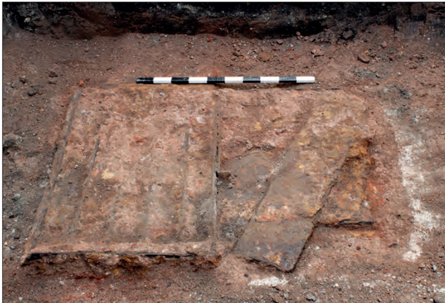
Figure 67: Iron capping over access hole into underground flue (group 1084) in coal store, looking north-east. Scale: 1 m (photograph by C. Mason).
