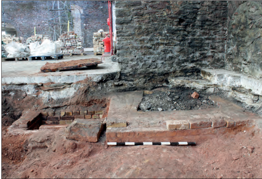
Figure 72: Openings at north end of flue (group 1084) in coal store, looking north-west (photograph by C. Sabato).
