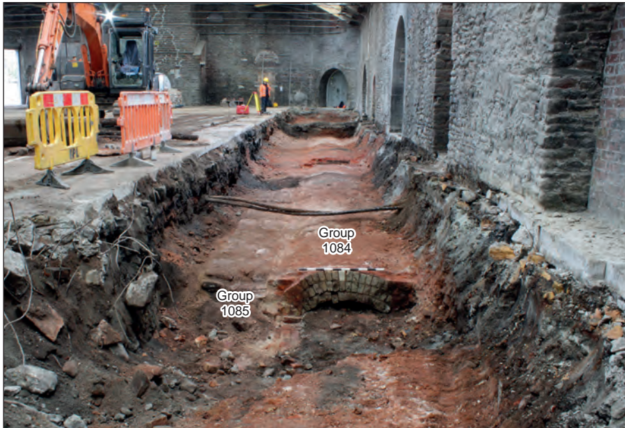
Figure 42: Stone wall foundation (group 1085) and brick flue (group 1084) in coal store, looking north-east. Scale: 1 m (photograph by C. Mason).
