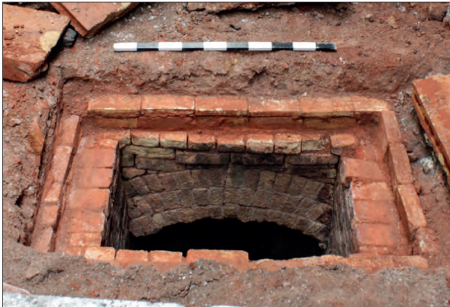
Figure 69: Access hole into underground flue system (group 1084) in coal store, looking north-east. Scale: 1 m (photograph by C. Mason).
