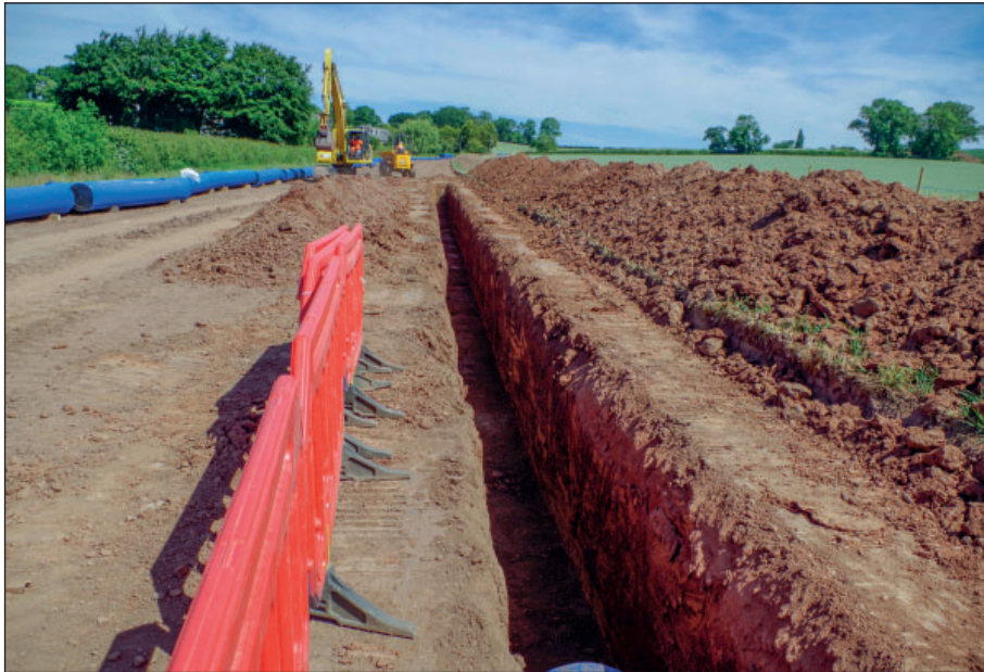
Figure 4: Topsoil strip and service channel, east of Chapel Lane, towards north end of stripped area, view from south
