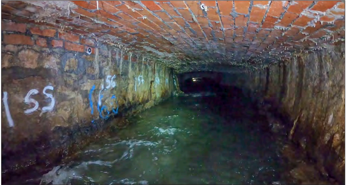
Photograph 21: The culvert to the west of the bifurcation (55m chainage)
