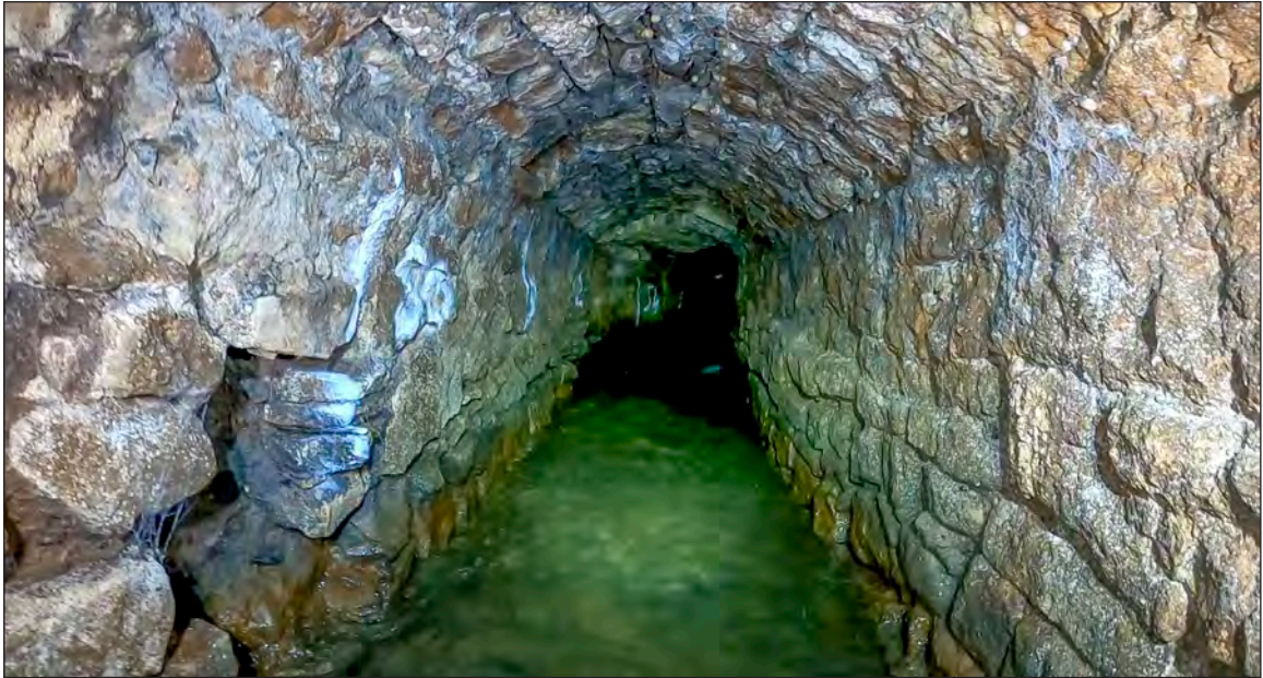
Photograph 19: Bifurcation left (49m chainage)
