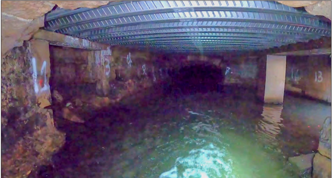
Photograph 8: The junction chamber viewed from the east
