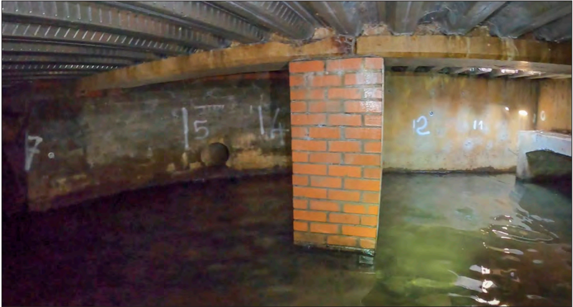
Photograph 9: The north side of the junction chamber, built in 2010.
