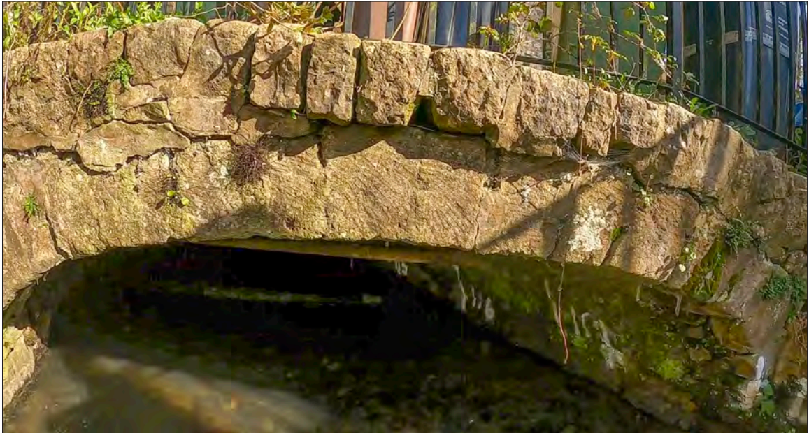
Photograph 32: The arch at the western end of the culvert (118m chainage)
