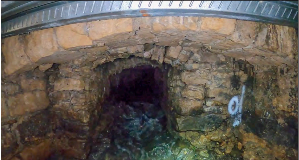
Photograph 7: The opening of the southern channel into the junction chamber
