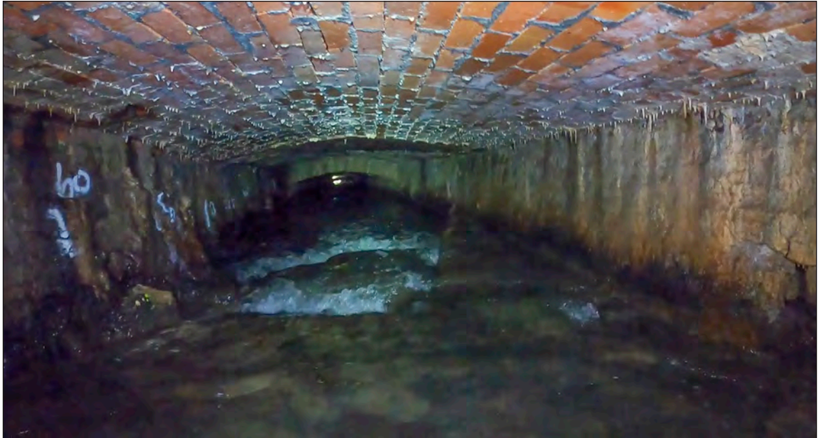
Photograph 22: A pair of drop structures lower the floor level (c.59m chainage)
