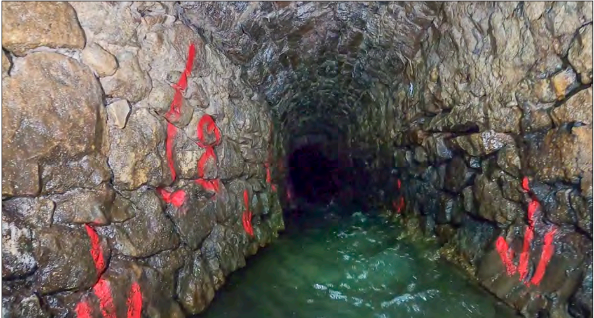
Photograph 4: Rough-coursed stone arch along the southern channel from the inlet
