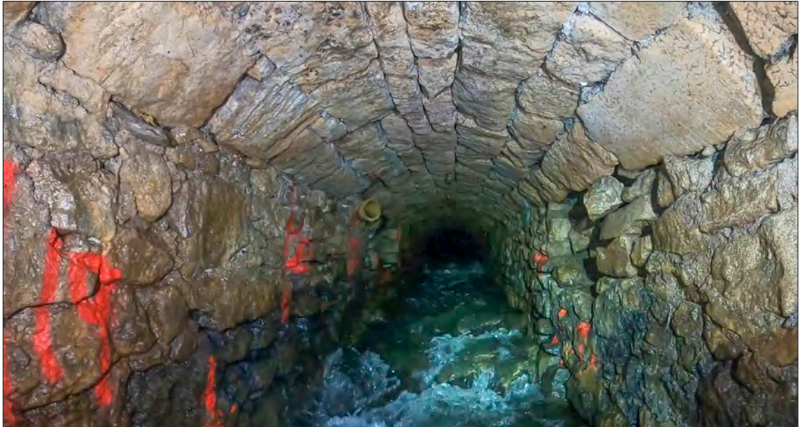
Photograph 2: Intact stone arched part of the southern channel from the inlet
