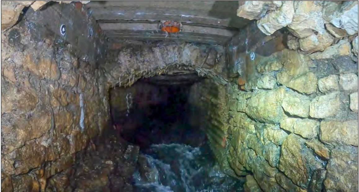
Photograph 6: The concrete soffit at the eastern end of the southern channel
