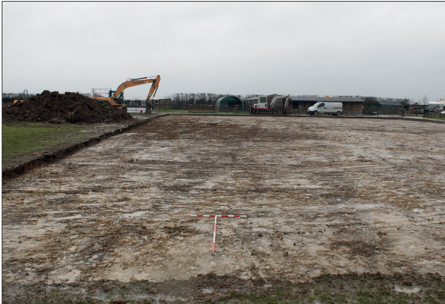
Plate 4: View of excavated area from east (2 m and 1 m scale)
