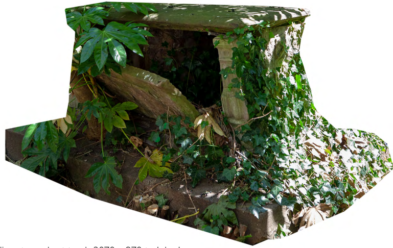
limestone chest tomb 2070 x 970 to John Jones dated 1785, with cement covered plinth
