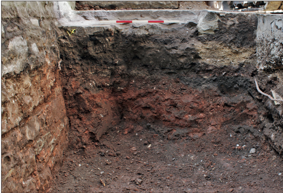
Figure 7: Representative section of deposit sequence below John Street, looking south-west, scale: 0.5 m (photograph by C. Hambleton)
