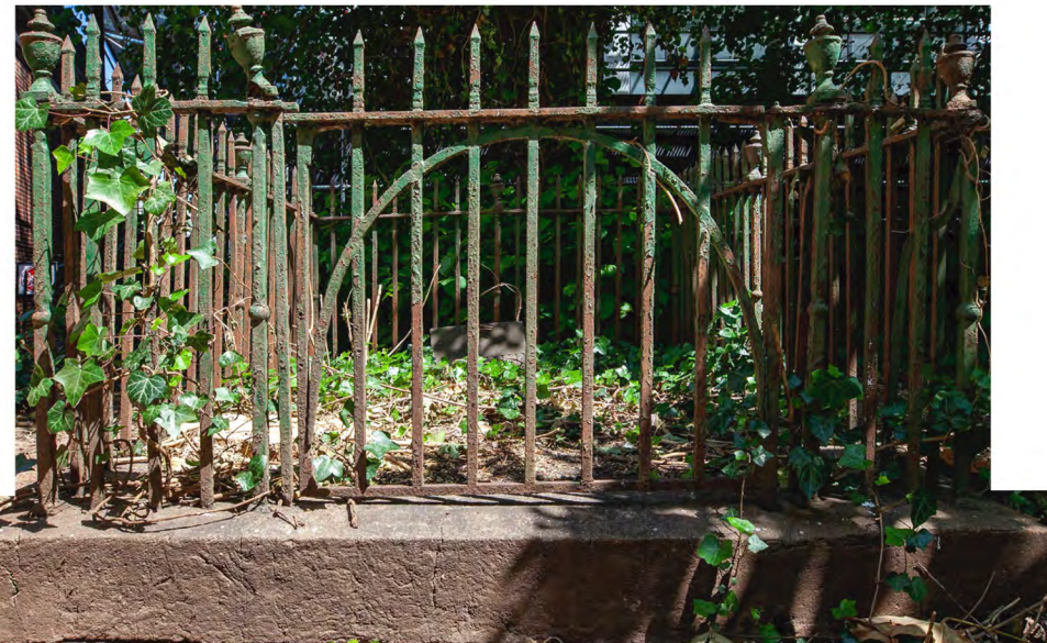
remove cement capping from stone plinths
