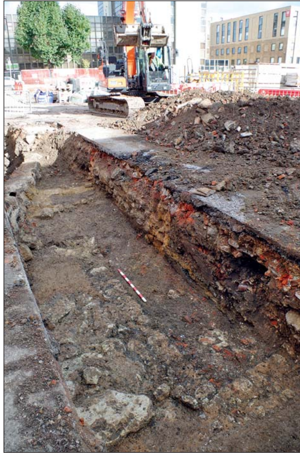
Plate 7: West 'arm' of trench 11, structural remains 1103–1108 exposed, from south-west (scale = 1 m)
