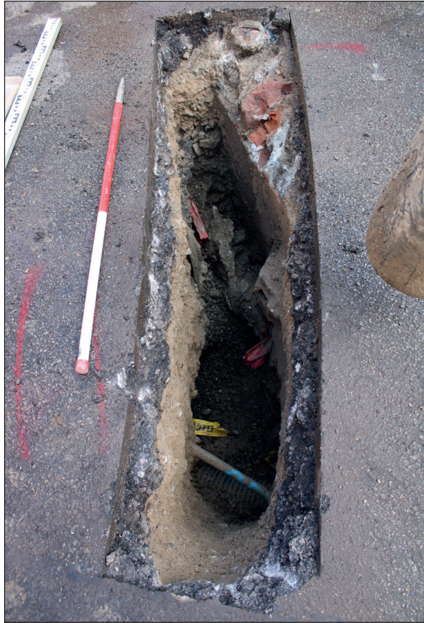
Figure 4: Slip trench 3, 1 m scale
