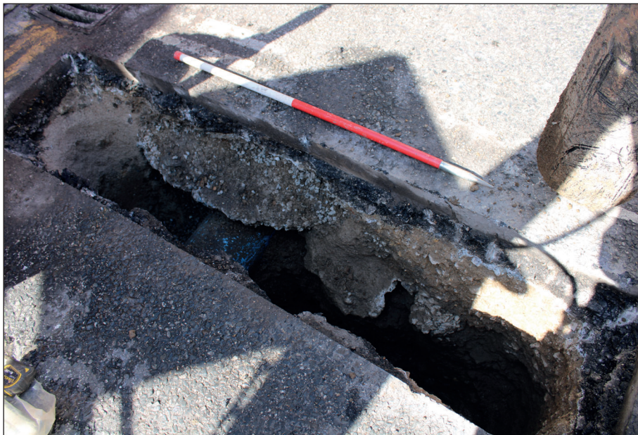
Figure 5: Slip trench 4 from the south-east, 1 m scale
