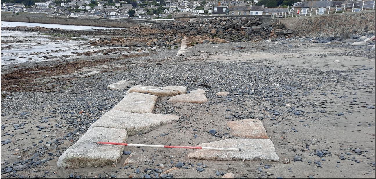
Figure 3: Granite kerb stones from old Newlyn to Penzance road. Access route runs through gap in centre of image
