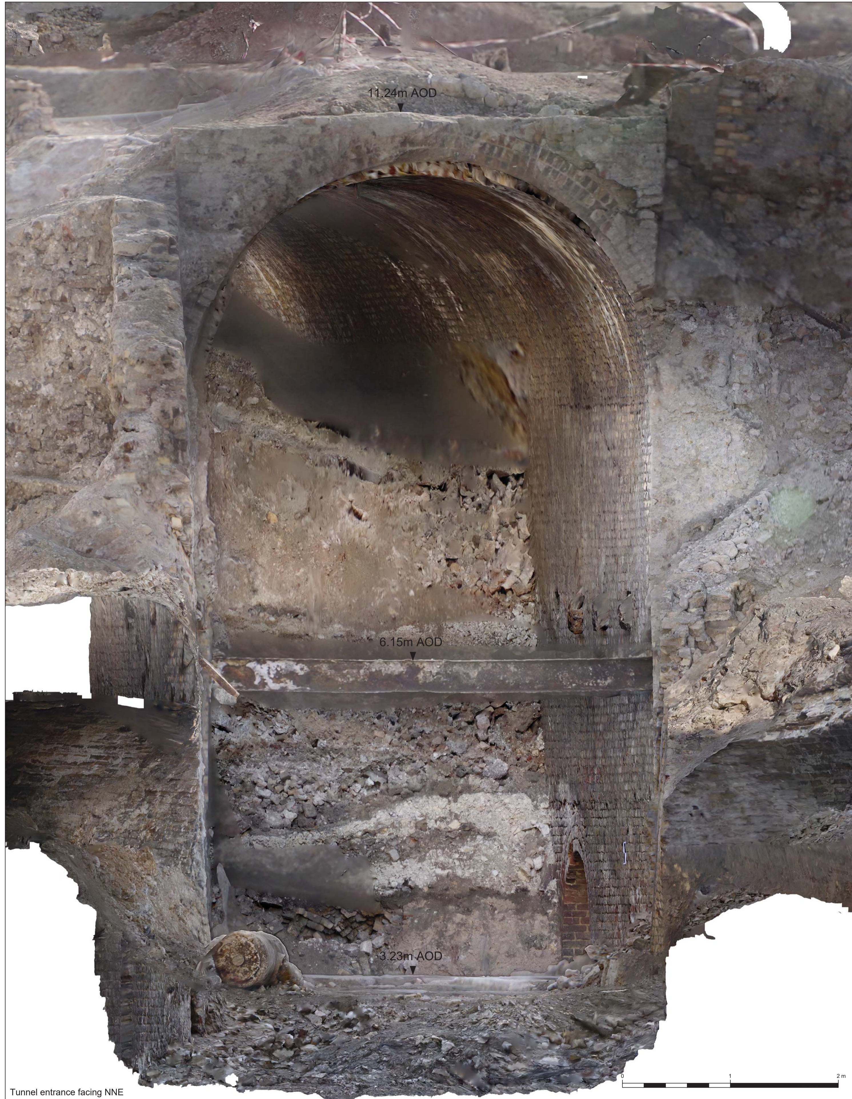
Tunnel entrance facing NNE
