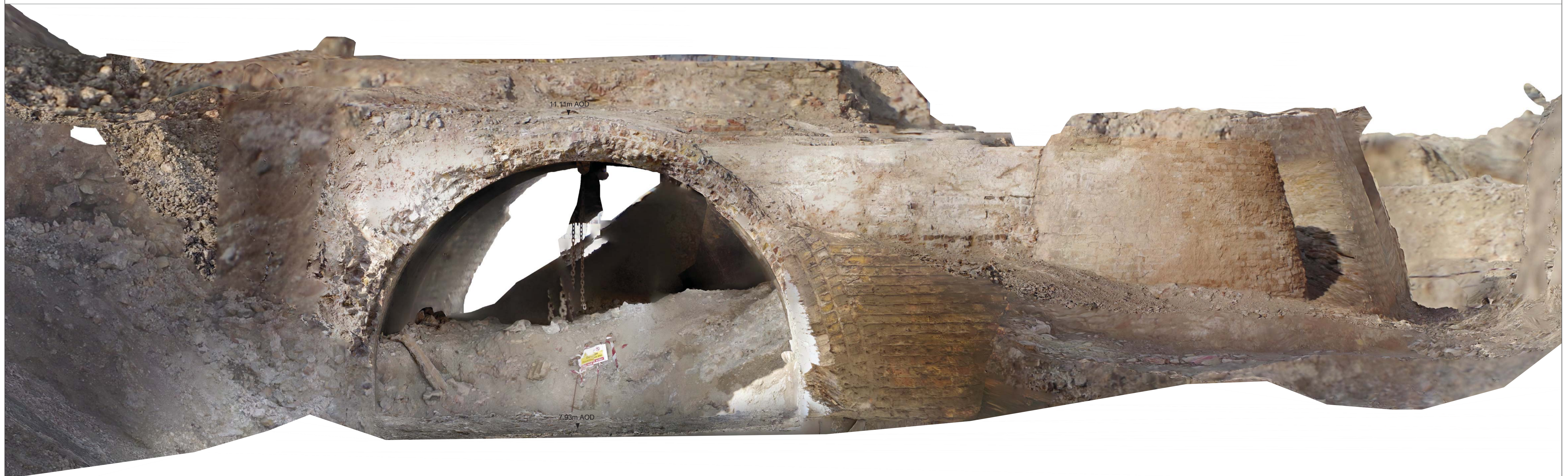
Southern tunnel entrance facing SSW
