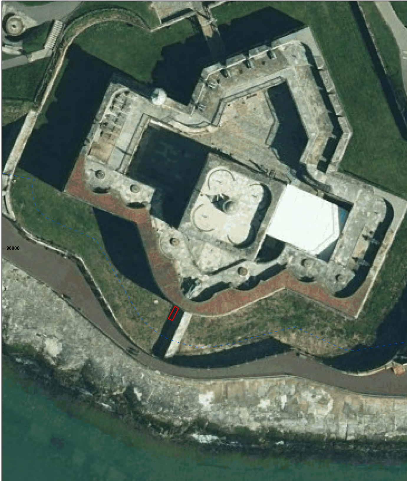
Location of monitored test pit
