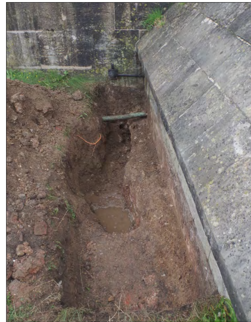
Photo 2) Interior castle wall 5807 and foundation 5808
