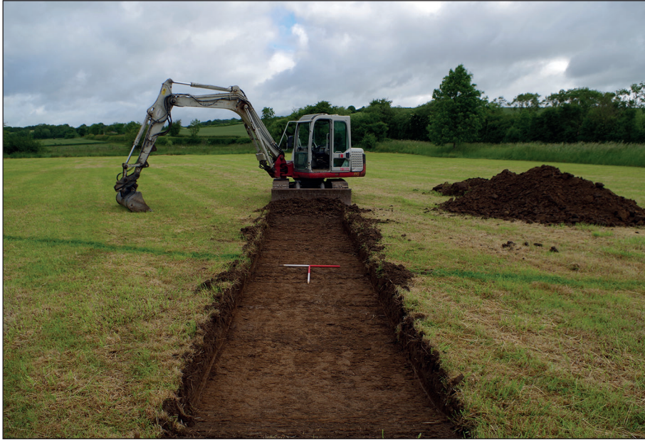
Figure 2: South facing view of excavation for the culvert (2 x 1 m scales)
