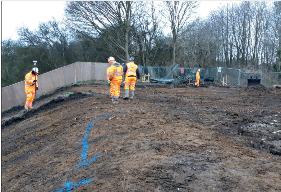
Figure 8: Trench 22 from the east (photographed by S. Froud)
