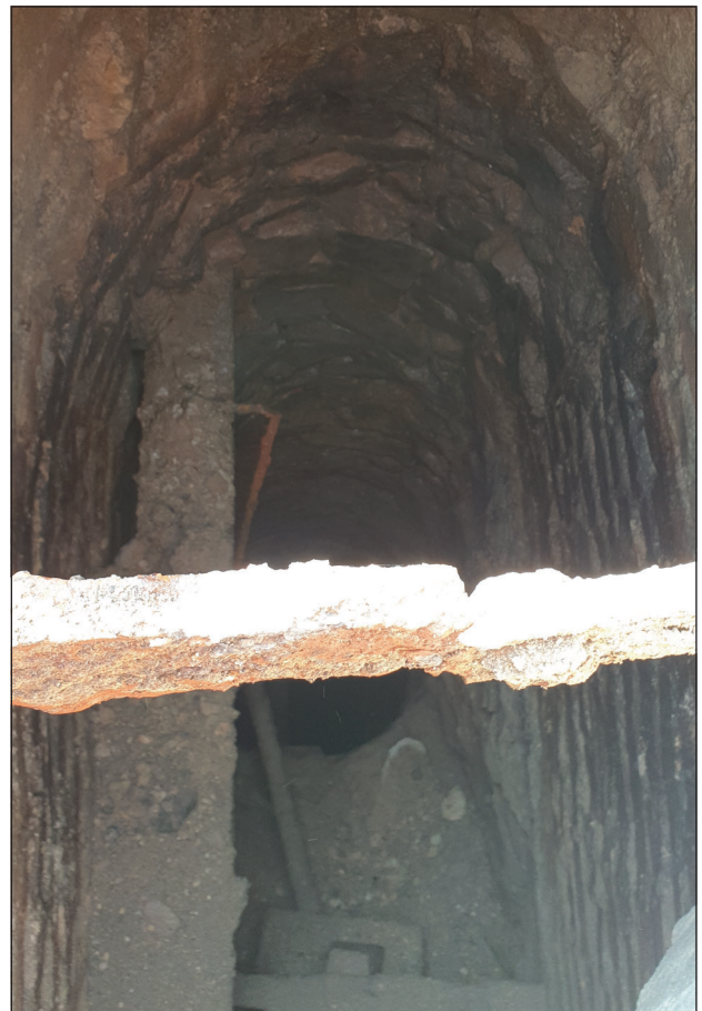
Figure 13: Well/pump 2402 and 2405 from the east (photographed by E. Troake)
