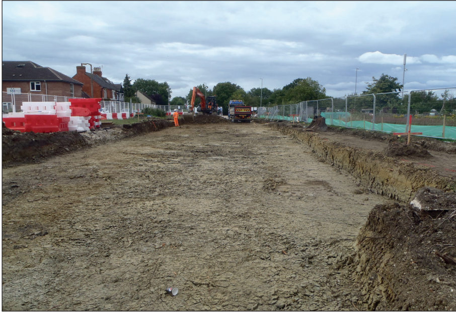
Figure 2: Trench 1 from the south-east (photographed by N. Fitzpatrick)
