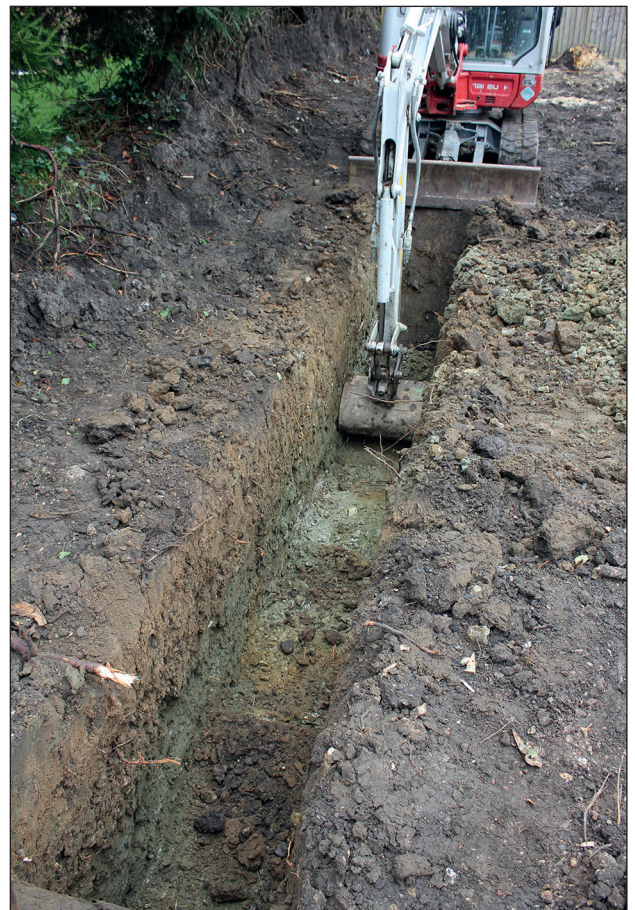
Figure 5: Working shot of south trench
