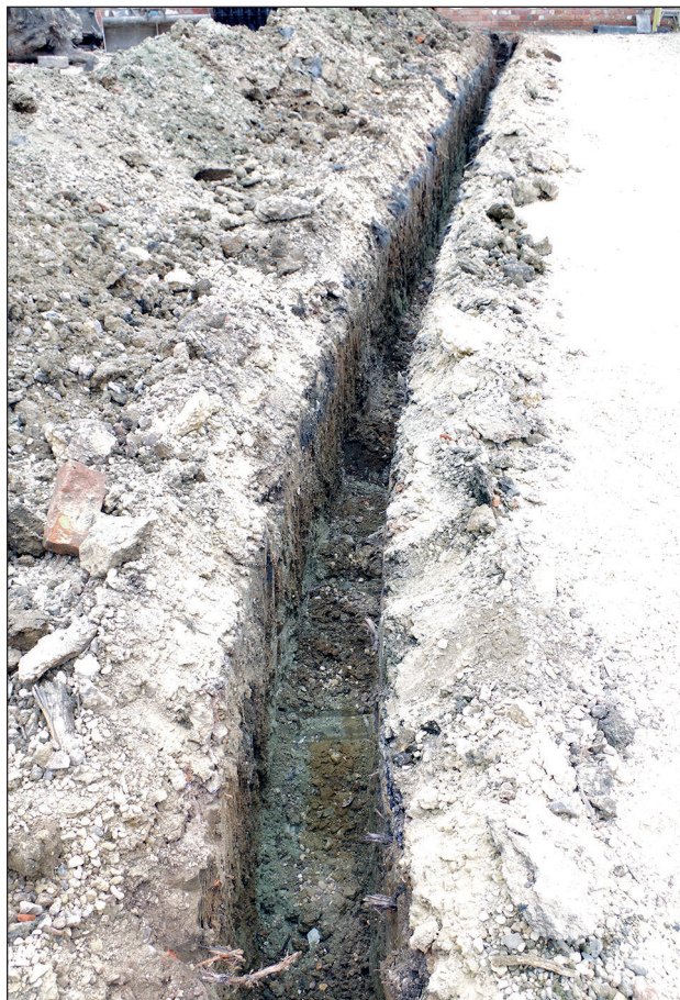
Figure 9: View of the southern part of the utility trench
