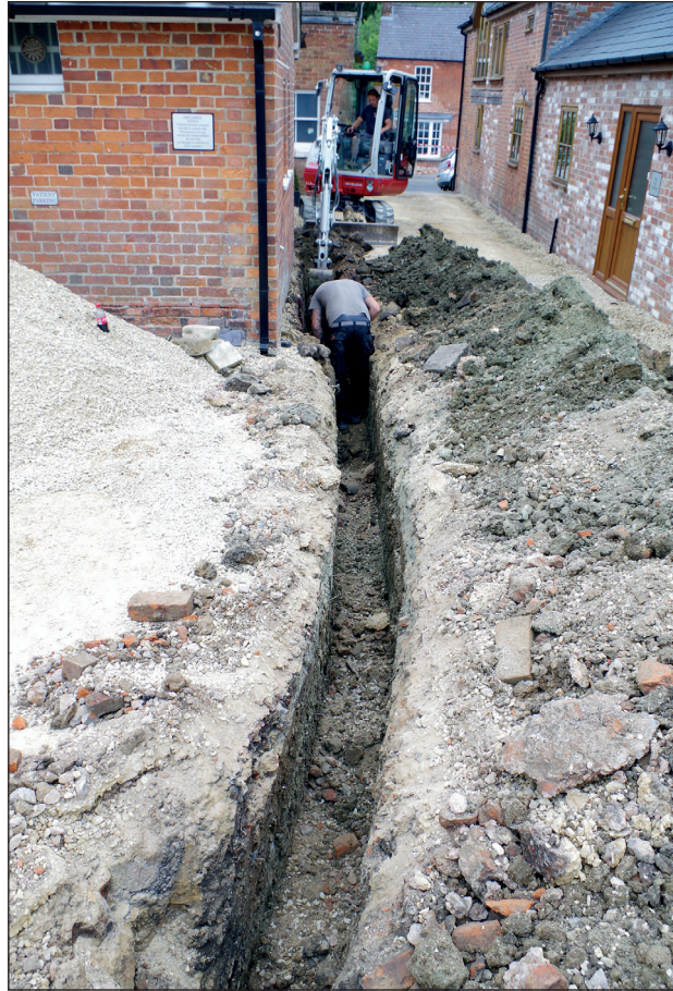
Figure 10: View of the northern part of the utility trench
