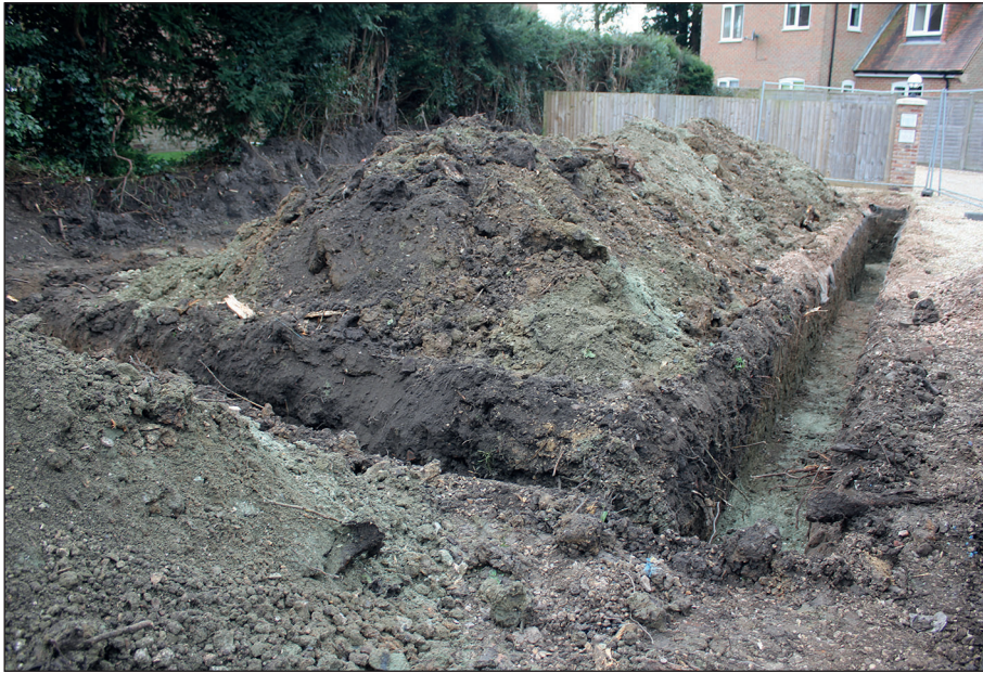
Figure 2: View of the completed footings from the north-east
