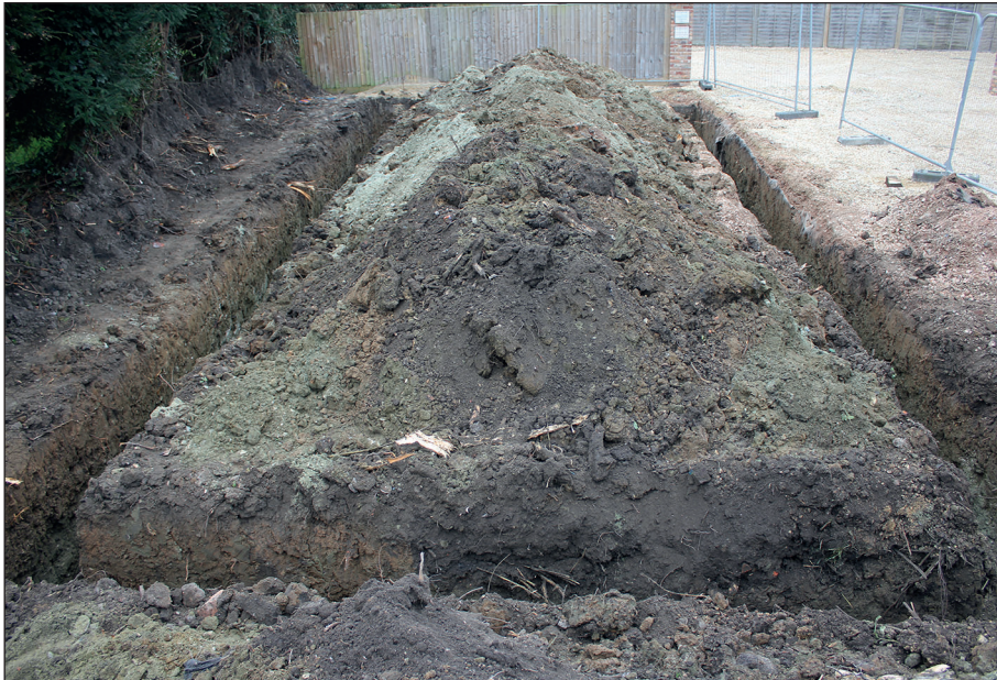
Figure 3: View of the completed footings from the east
