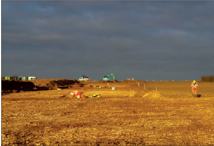
Figure 132: Area 5, working shot of area strip, view from the south-west
