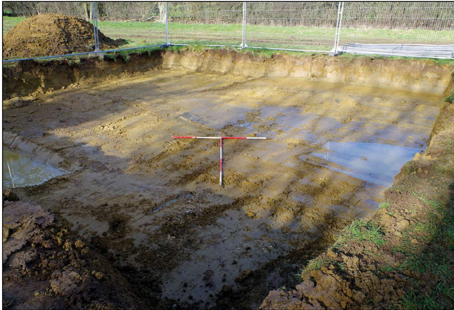
Plate 21: Area 6 from the south (scales: 2m)
