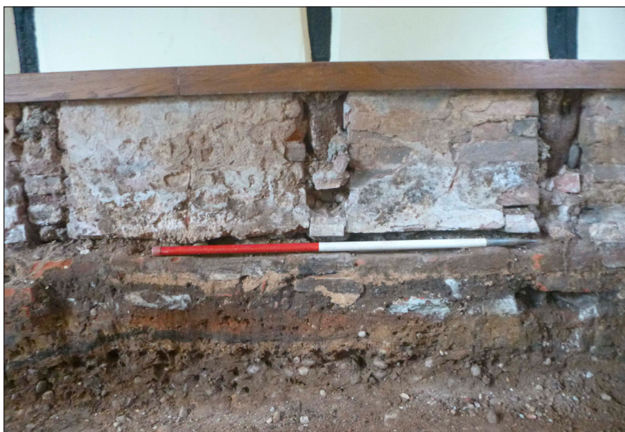
Figure 9: Close-up of layers 108–112 and possible brick floor 161 beneath internal wall 107/159, viewed from the south-east, 1 m scale.
