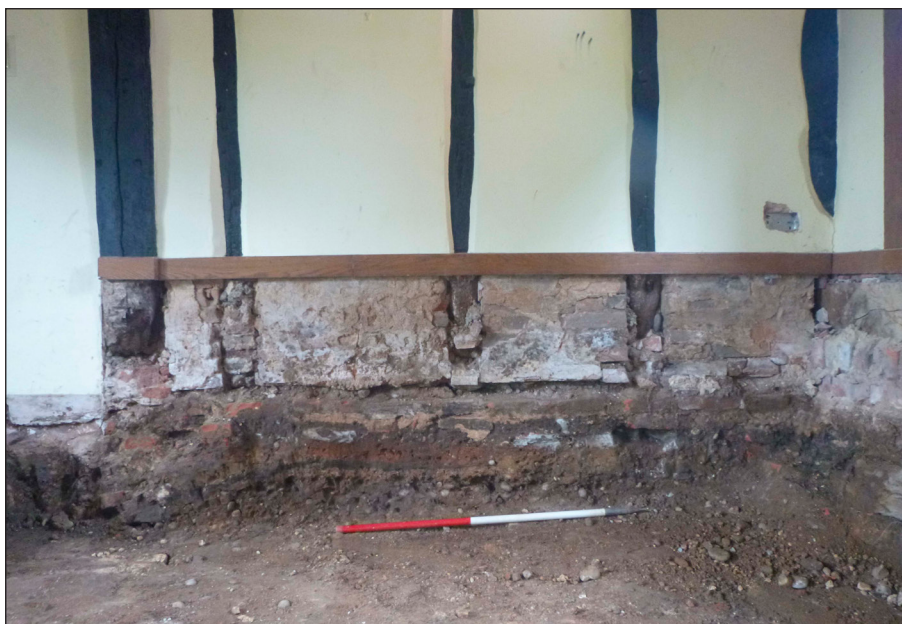
Figure 8: South-east facing internal wall 107/159 of main building, 1 m scale.
