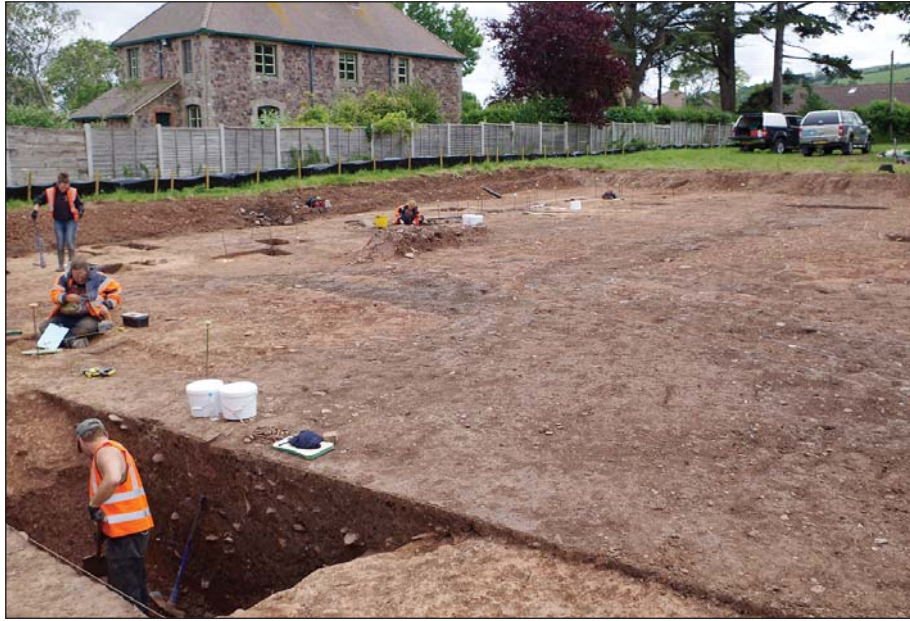
Plate 1: Working shot of Site from the north-west, with ditch 301 in the foreground
