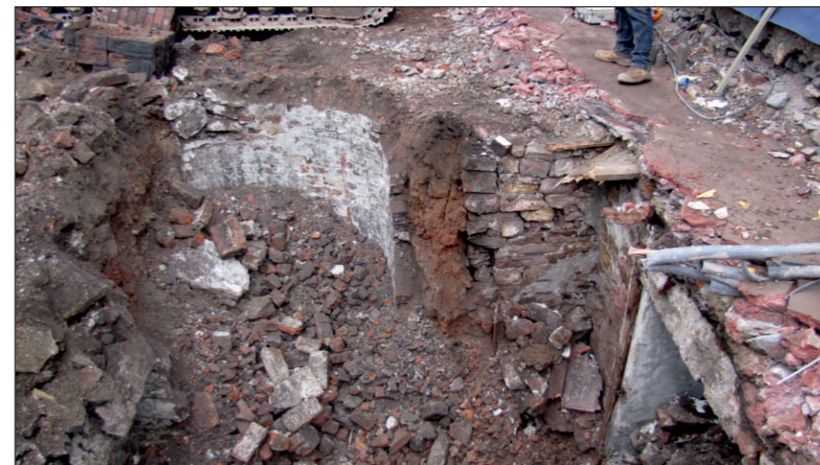
Plate 17: Detail of curving passage 1912 during demolition from south
