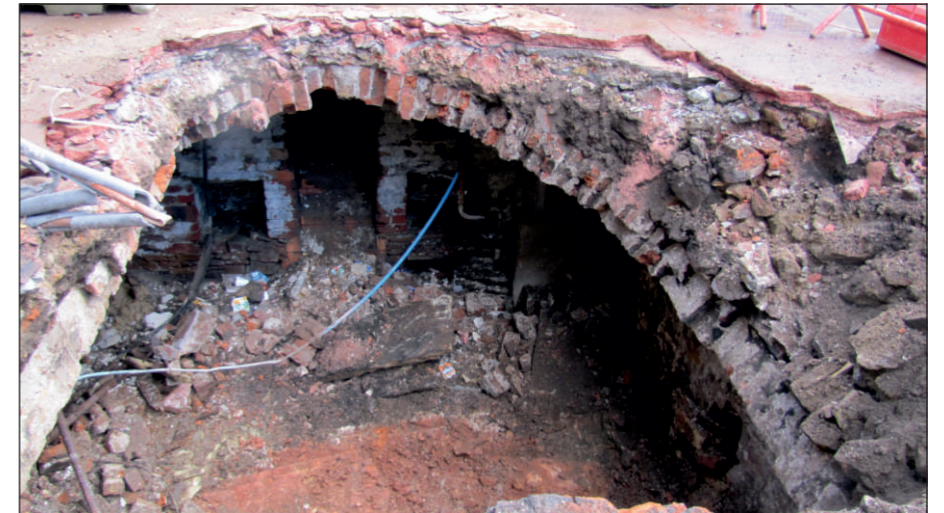
Plate 15: Watching brief trench 19 from north showing wall 1906 under vaulting 1900
