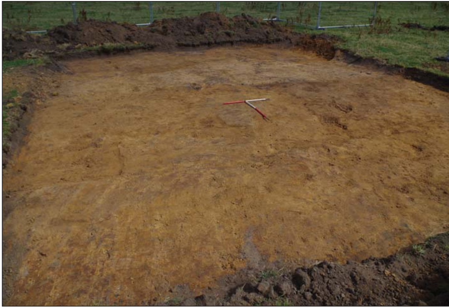
Plate 7: View of open area excavation from the south-west
