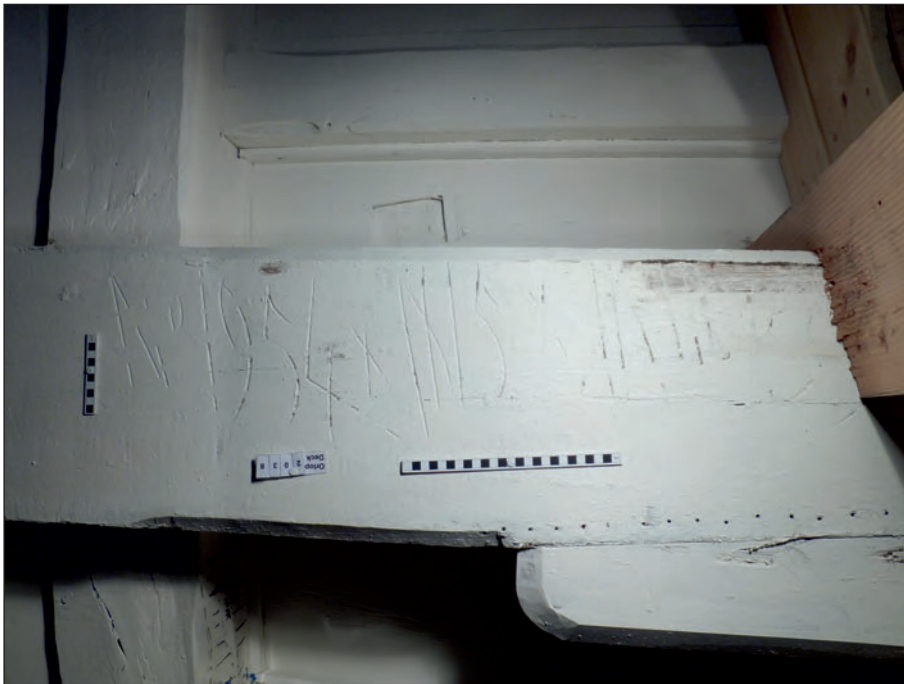
Plate 5: Typical 1815 rase mark syntax, Timber Mark 2038
