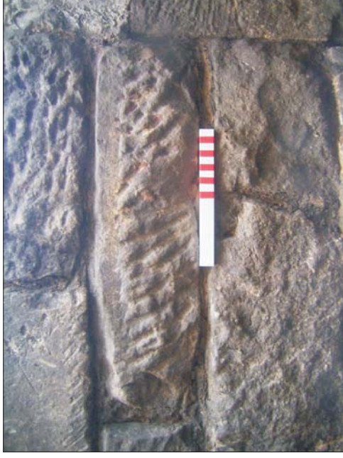
Plate 6: Roman stone block re-used in the west-facing elevation of Victorian cellar entrance chamber 110
