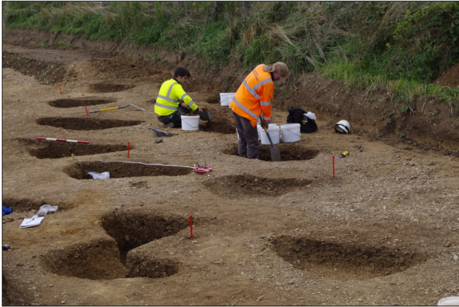
Plate 11: Working view of the excavation of pits in Area 6, viewed from the north-east (1 m scale)
