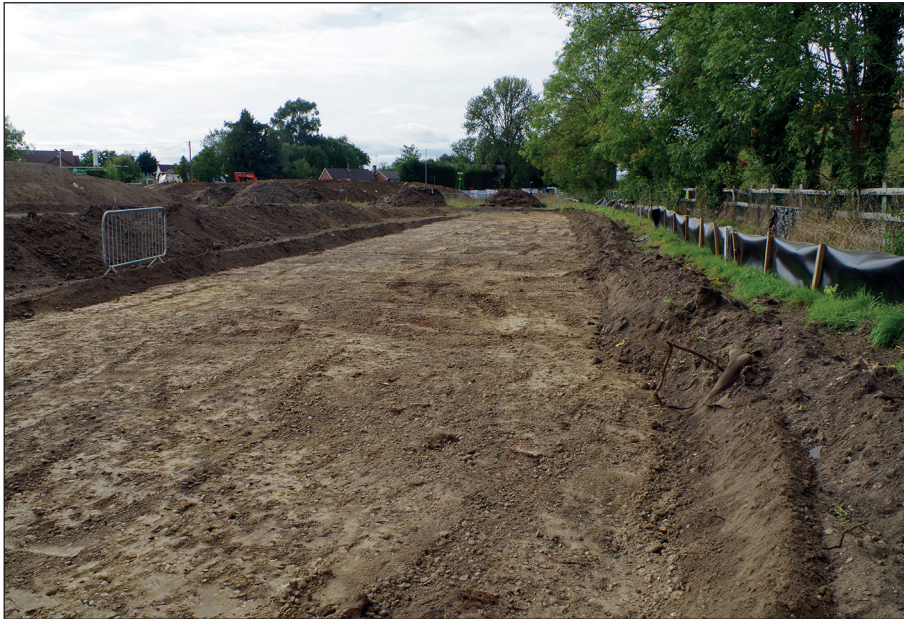
Plate 3: Northern edge of Area 1, view from the east.
