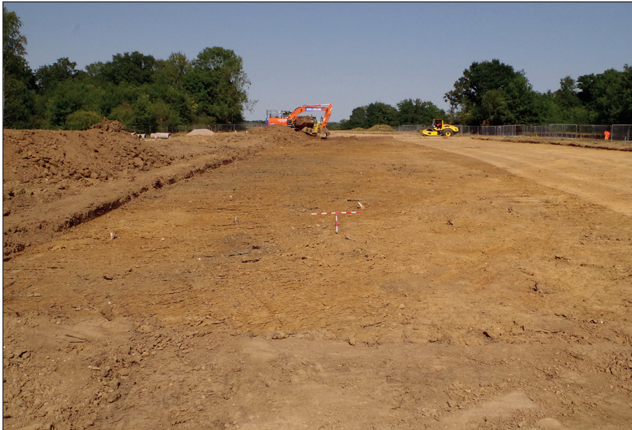
Plate 2: Stripping of Area 3. 1 m and 2 m scales.
