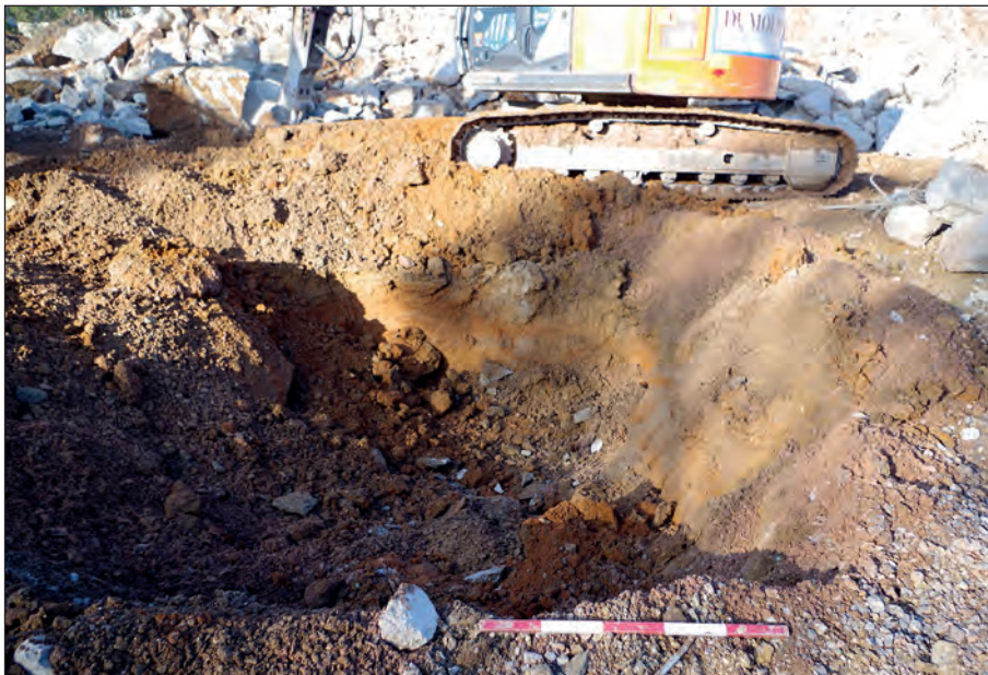
Plate 14: Trench 19, viewed from the south. Scale is 1 m
