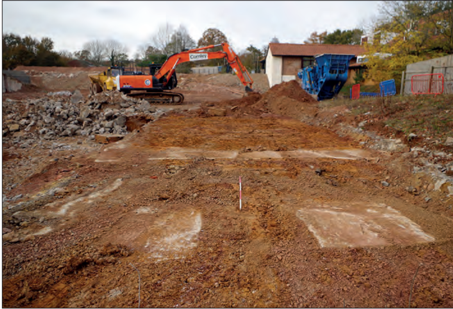
Plate 17: Trenching, north-west area, viewed from the south. Scale is 2 m
