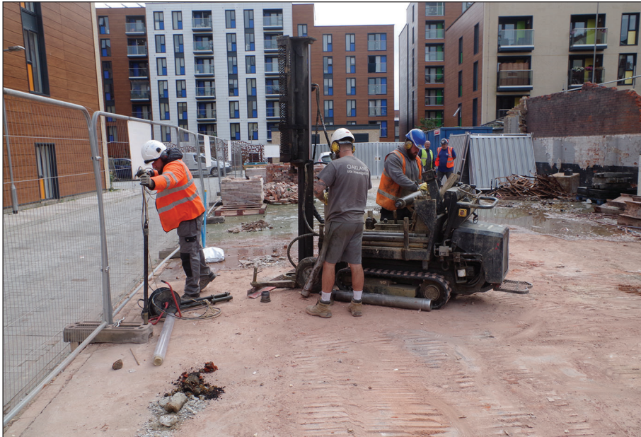
Plate 4: Working shot showing Window Sampling at WS02. View from West
