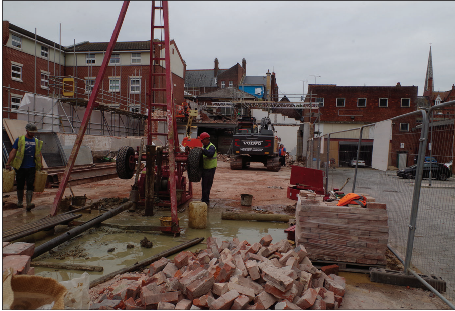
Plate 1: Working shot of Cable Percussion Drilling (Trench 10/BH01) – View from East
