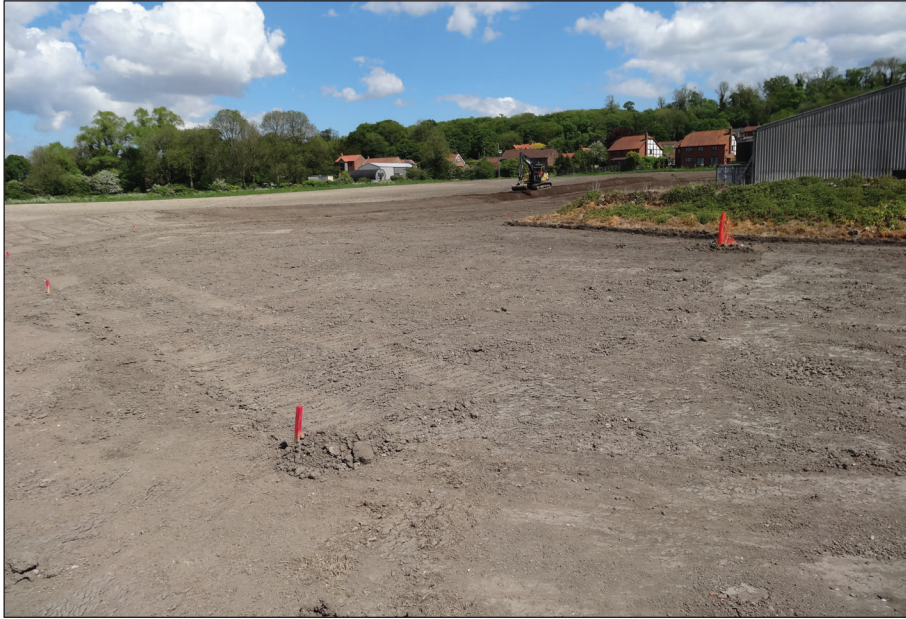
Plate 3: WB area 2 stripped (view from SW)
