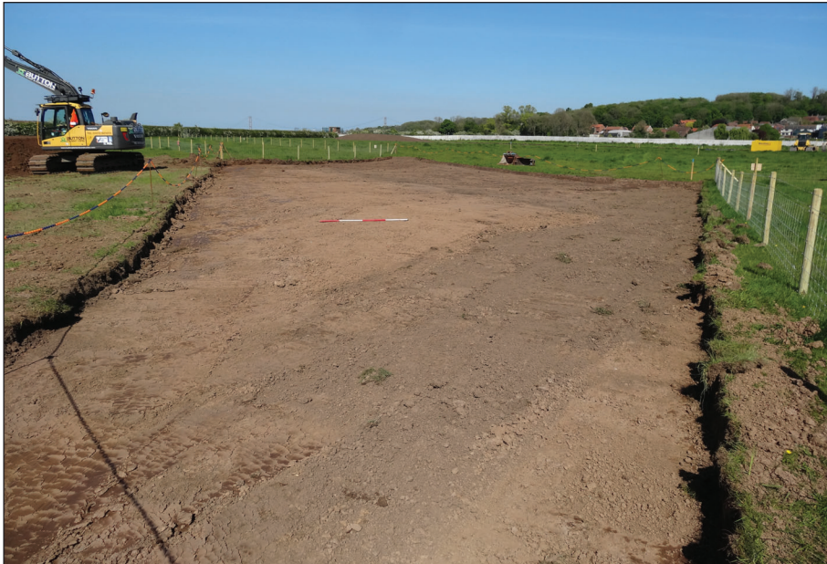
Plate 2: WB area 1 stripped (view from SW)
