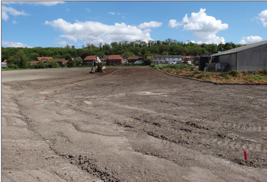
Plate 4: WB area 2 stripped (view from W)
