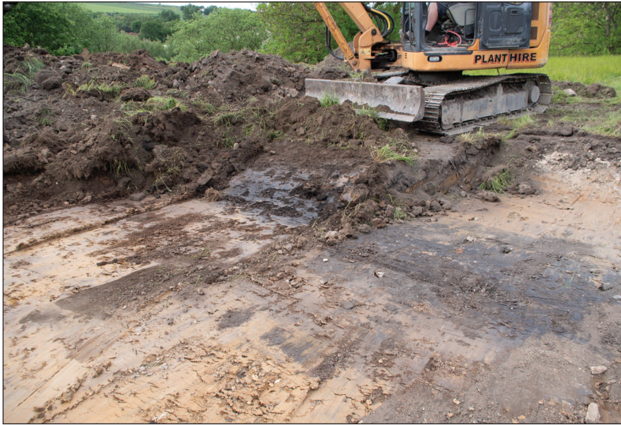
Plate 3: Working shot of excavation
