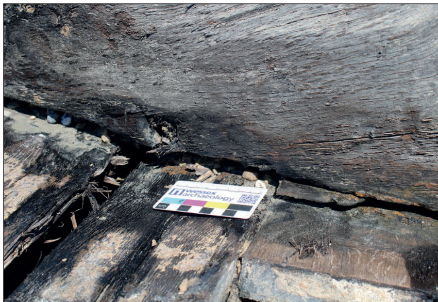
Figure 37: Small wedges were inserted underneath some of the frames
