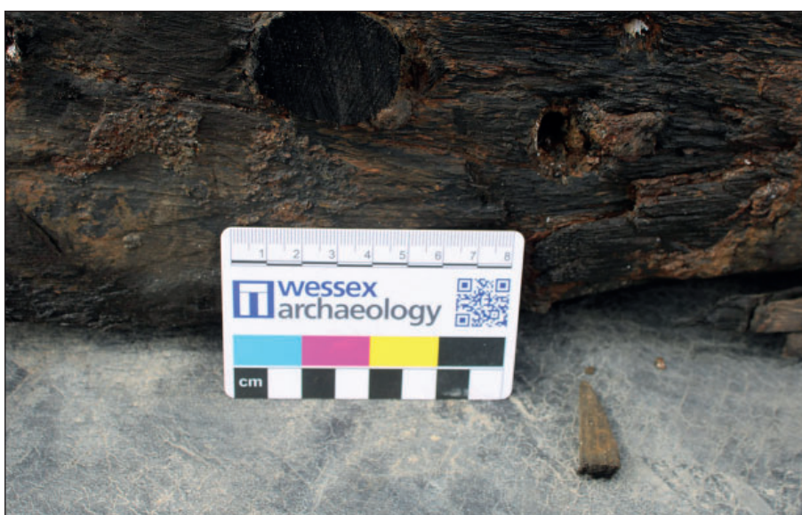
Figure 22: Small plug for temporary fasteners found on the underside of the frame [069]
