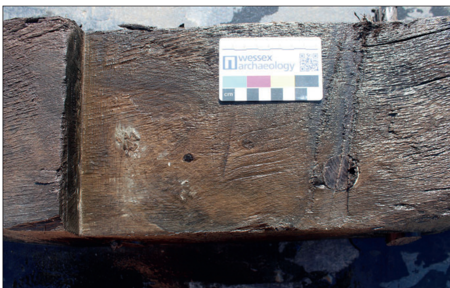
Figure 42: Possible marks seen on timbers
