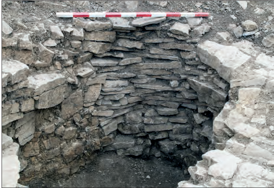
Figure 22: Dry stone wall revetment 5056, in pit 5054, from the north-west, scale 1 m (photograph by L. Newton)
