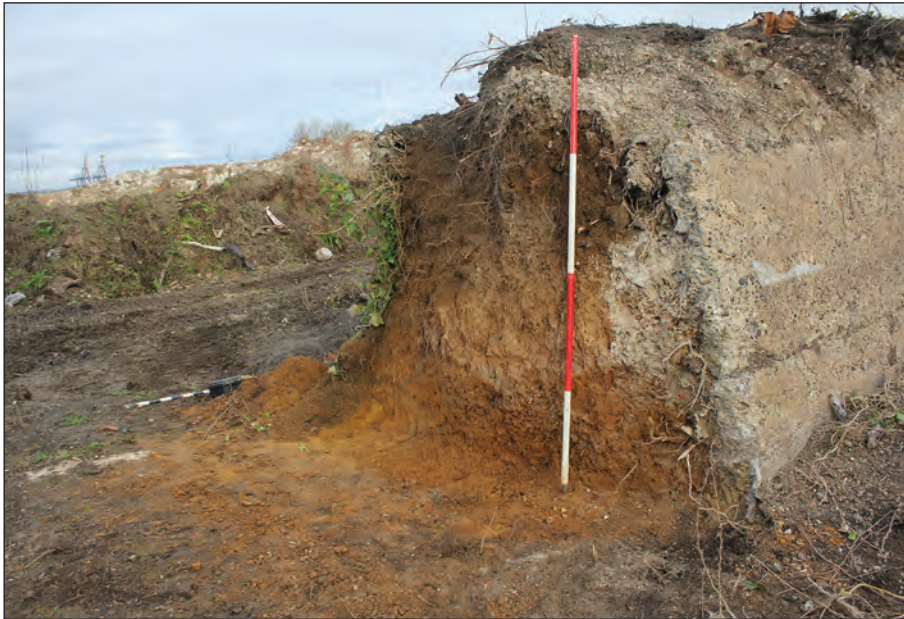
Plate 13: Breach in concrete wall of chalk slurry back, Sec 29, Area 3
