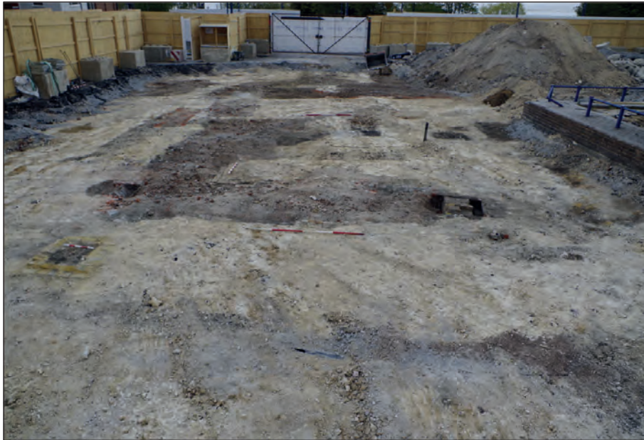
Plate 7: Irregular basement foundation 1240, viewed from the south
