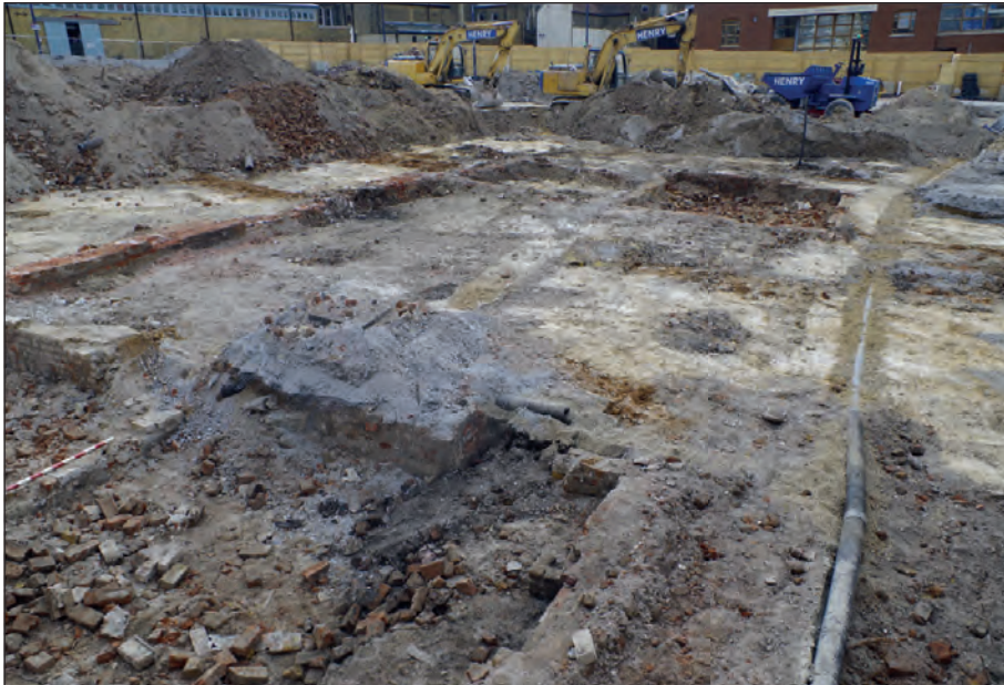
Plate 14: Boundary wall 1126, basements 1127 and 1129 and wells 1123 and 1124, viewed from the east
