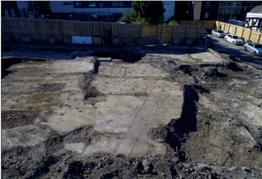
Plate 24: Courtyard on 'Bull Yard' routeway, viewed from the east
