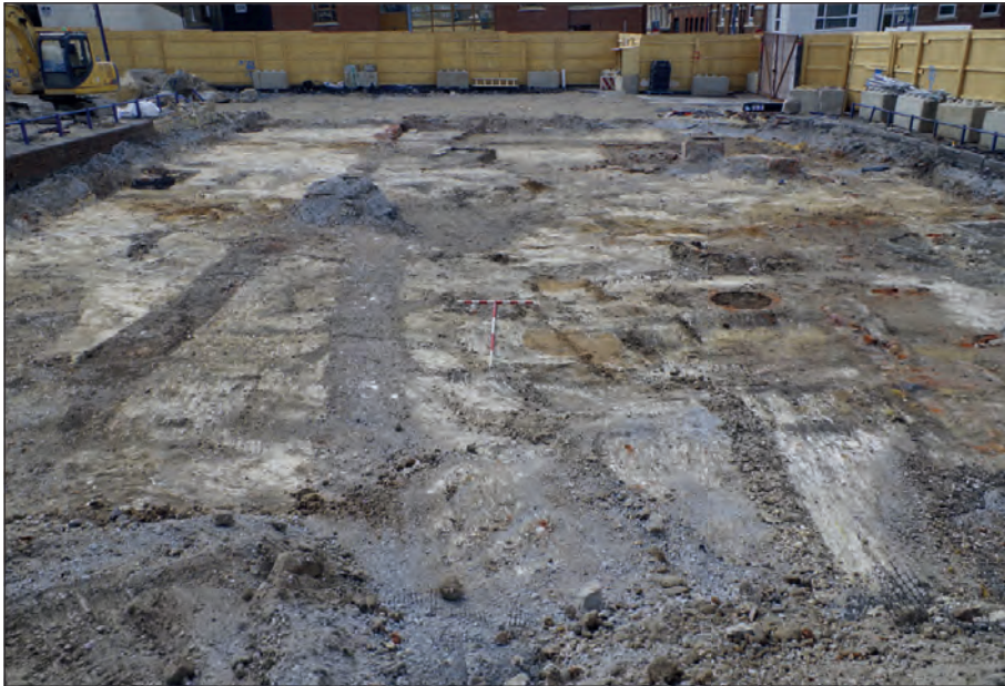
Plate 17: Northwest quarter of southern car park, viewed from the east
