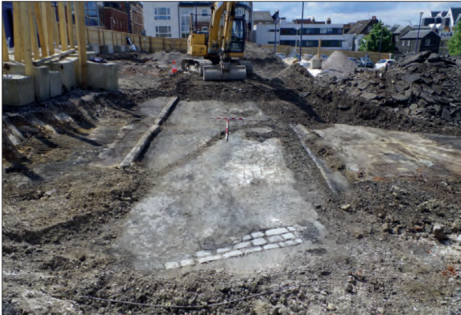
Plate 22: Eastern end of 'Horn Yard' routeway, viewed from the east
