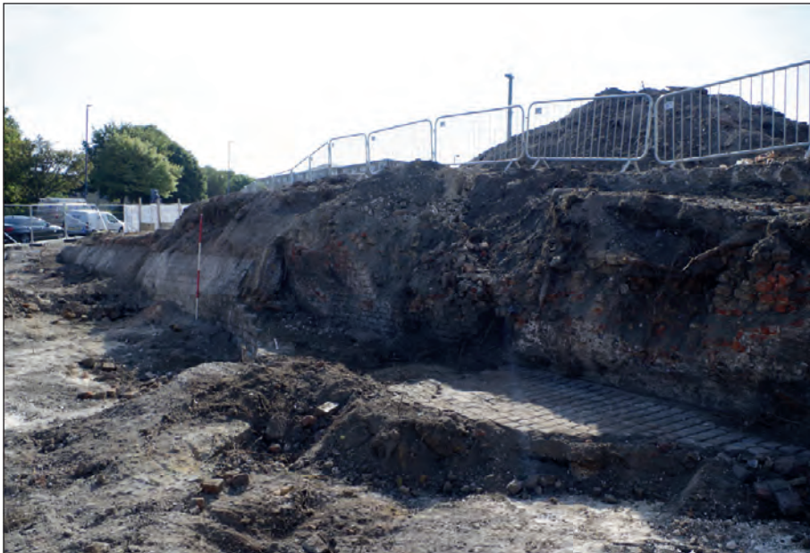
Plate 25: Retaining wall 1210, viewed from the northwest
