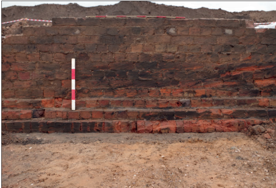
Plate 16: Wall 81 viewed from the north (0.5m scale)
