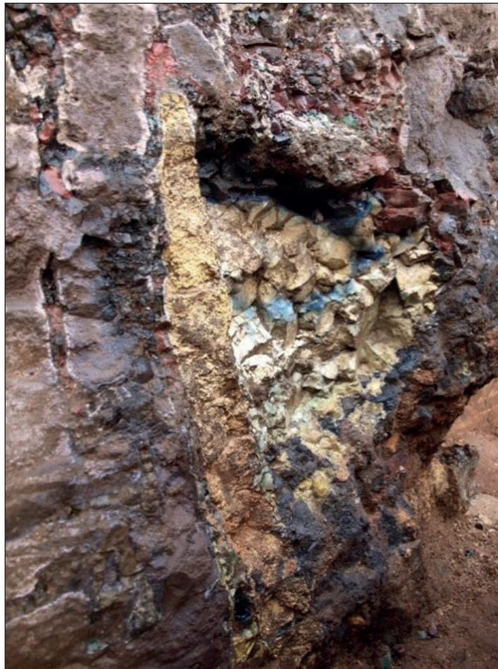
Plate 43: Photograph taken of the cut through the siege (south-facing section). This image shows the lower part of the siege, while Plate 42 shows the upper part. These two images demonstrate that the construction method used resembled an ashlar-and-rubble technique in which the 'ashlar' was refractory brick while the rubble core was composed of miscellaneous devitrified glassworking waste. This image also appears to show the reuse of a crucible
