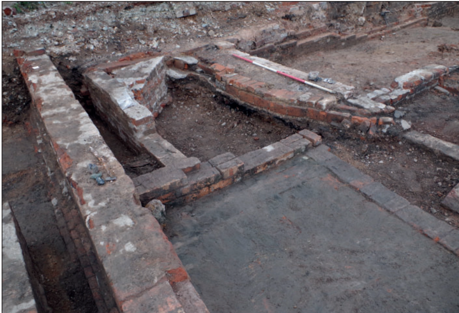
Plate 8: Room 501 with later floor 237 in the foreground, viewed from the south-west (2m scale)
