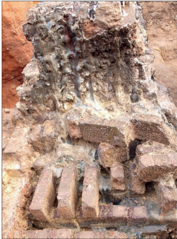
Plate 41: Photograph taken on the west side of the siege remains (looking east). The side of the siege (above the regenerator bricks) shows extensive vitrification and erosion of the siege by glass
