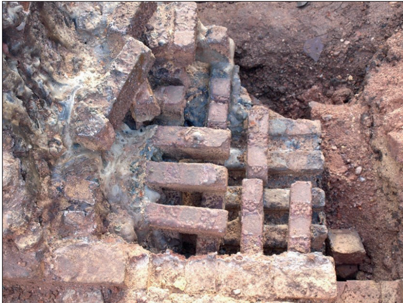
Plate 40: Photograph taken on the west side of the siege remains (looking south). This shows the regenerator bricks arranged in a chequer-board formation to ensure the through flow of air. The bricks have been preserved in position by a subsequent flow of glass (opaque white?) from the left (siege) side.
