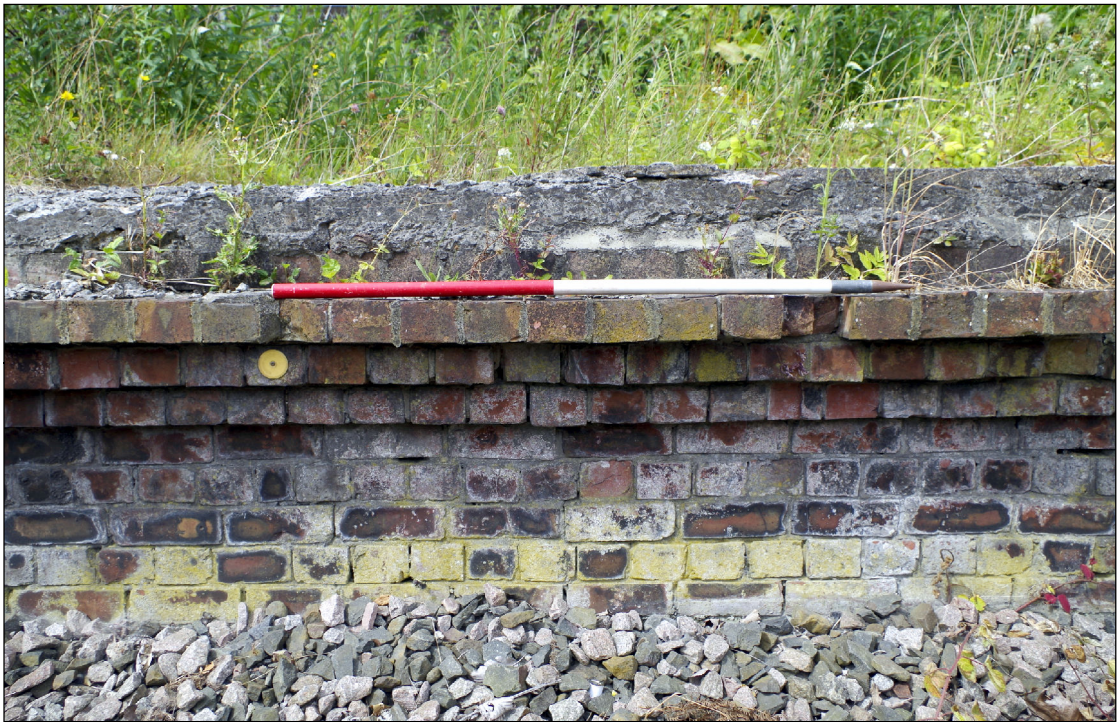
Photograph 3) View of the West Platform's northern section, facing west
