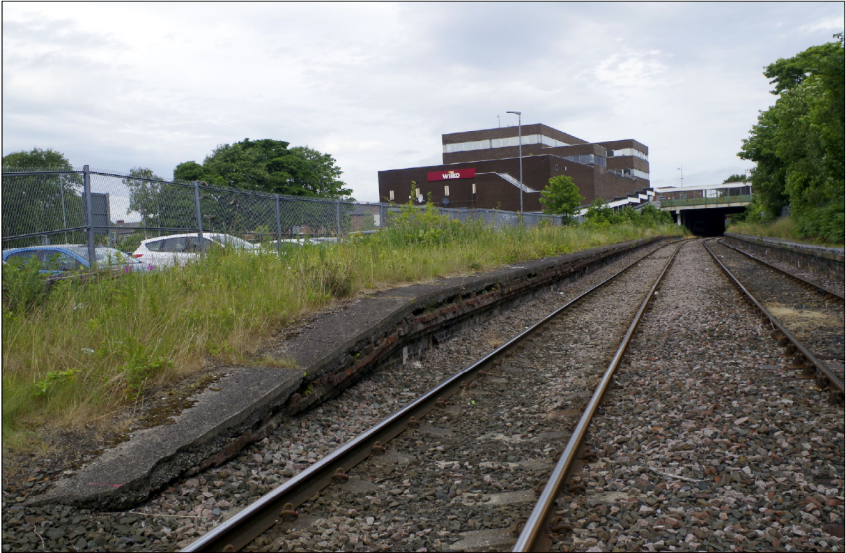
Photograph 1) View of the West Platform from its southern end, facing north
