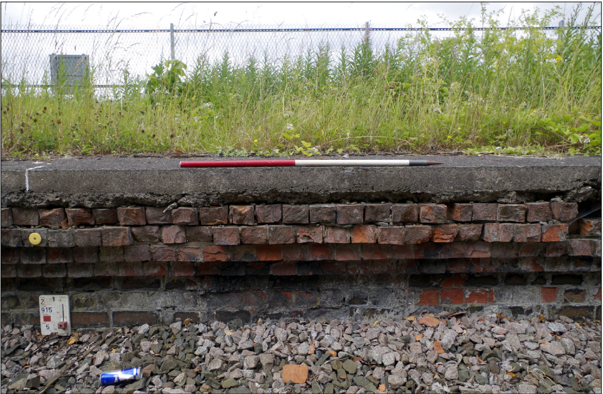
Photograph 2) View of the West Platform's southern section, facing west
