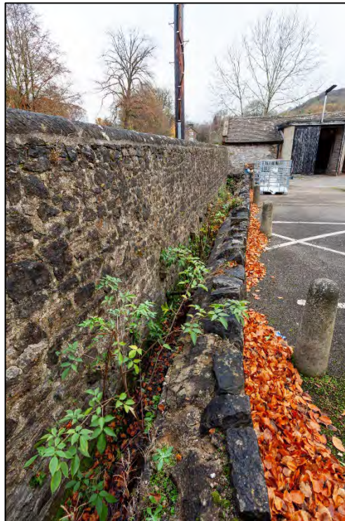
Plate 13: Canalised stream along the west side of the yard, facing north
