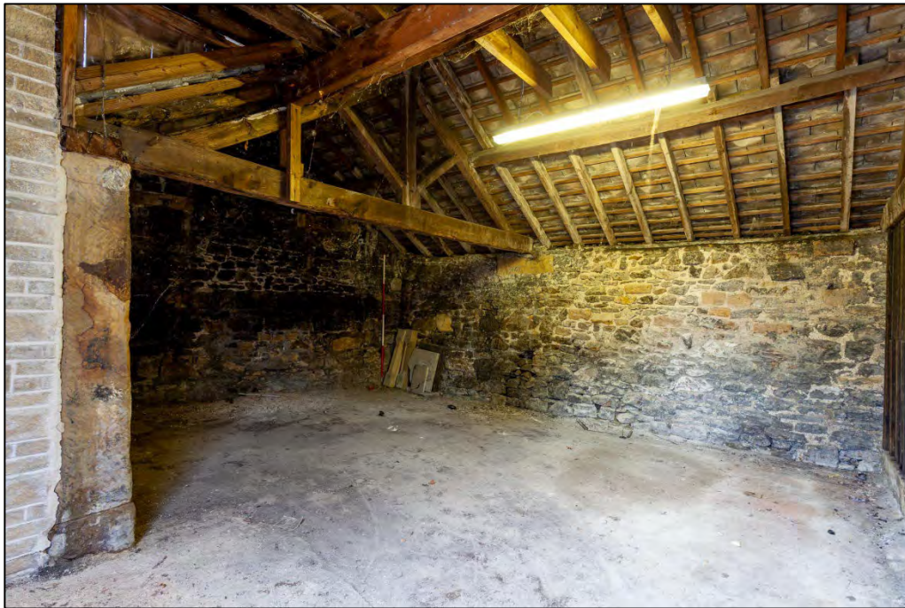
Plate 17: Western room of the Cart House, facing northwest
