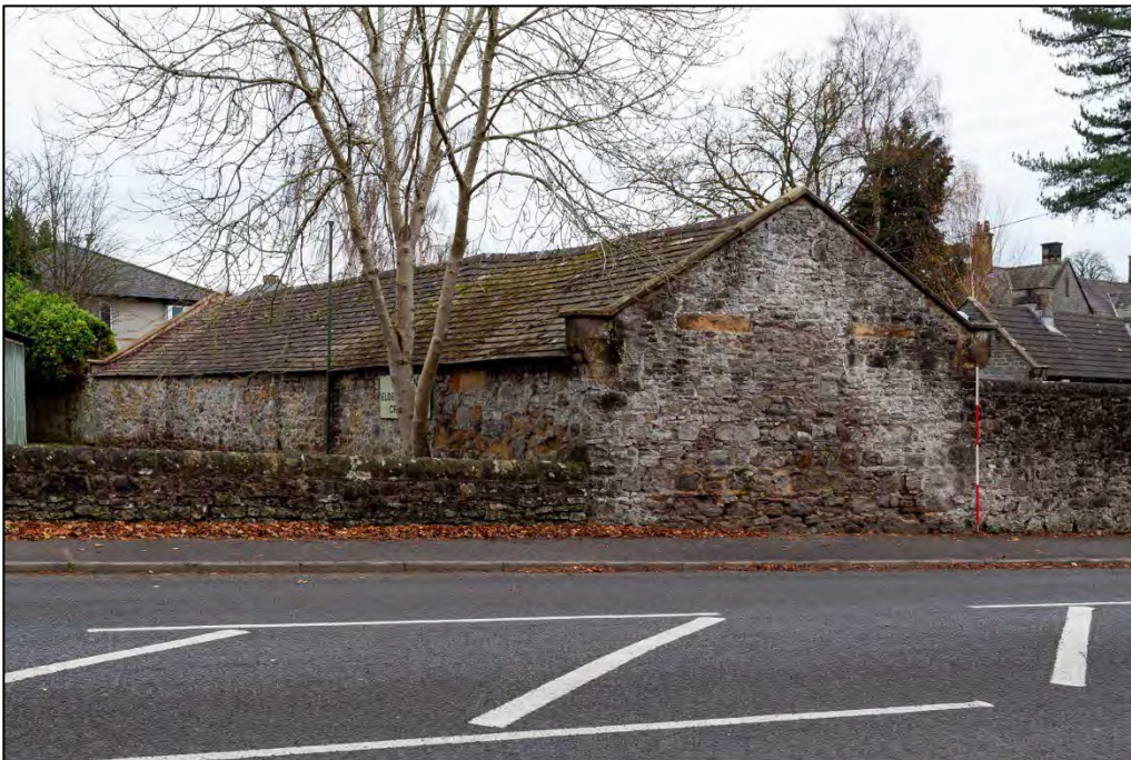
Plate 4: North and west elevations of the Cart House, facing southeast
