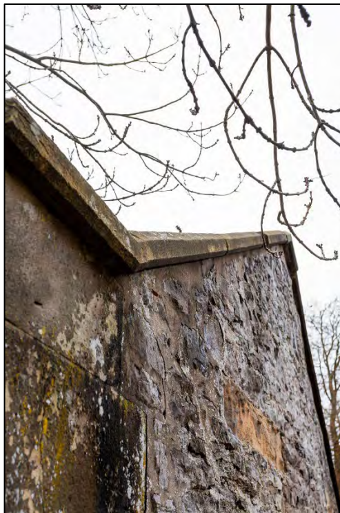
Plate 12: Detail of coping to the Cart House's western elevation
