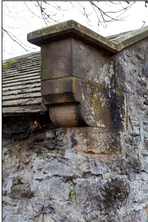
Plate 11: Detail of gritstone kneeler to the Cart House's western elevation
