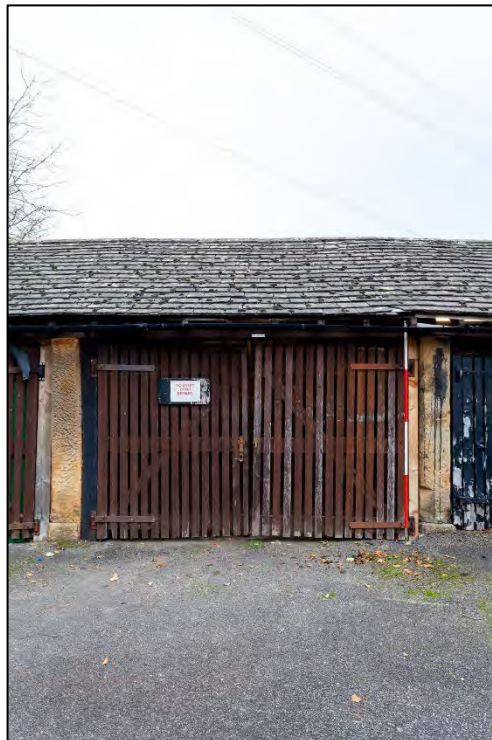
Plate 6: Gritstone columns and timber doors to the Cart House
