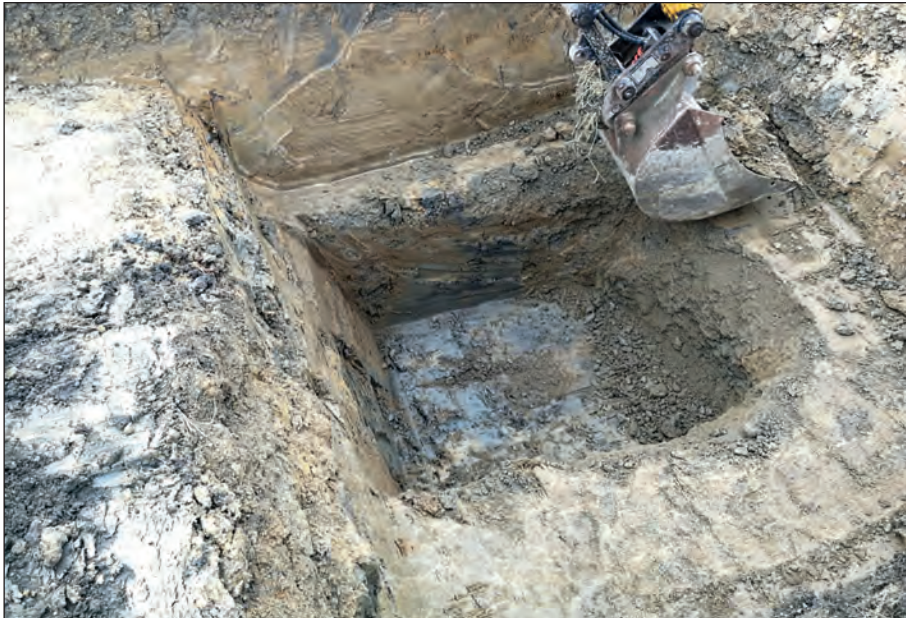
Plate 4: Excavation of shaft in northern area looking west
