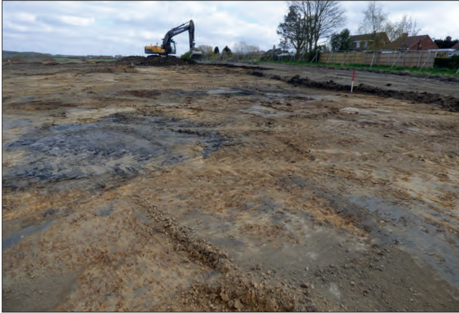
Plate 1: Southern watching brief area showing shafts, looking south east
